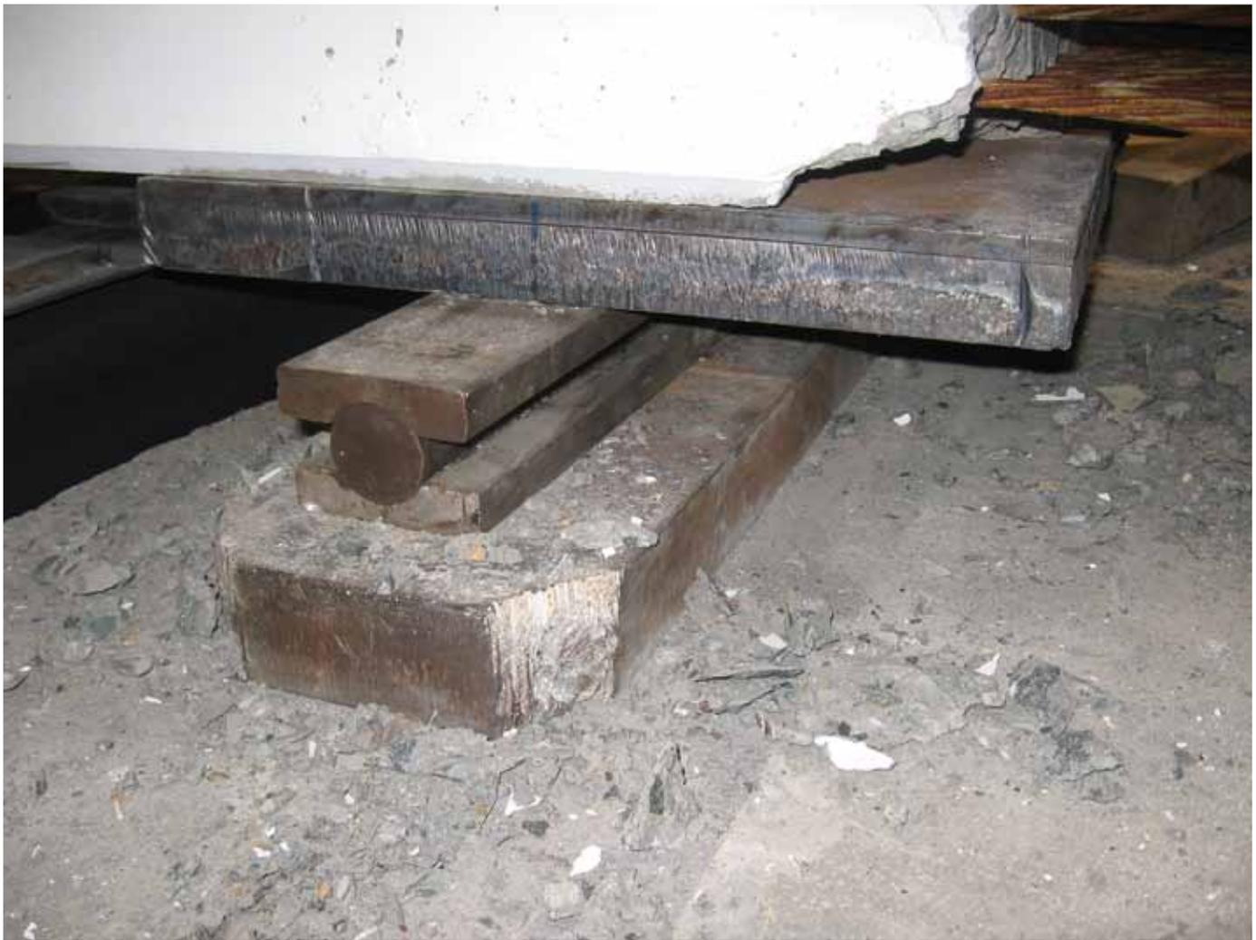
**Figure 8.** Pivoting support with a larger bearing area used for ends VA1L, VA2R, and VA2L.
