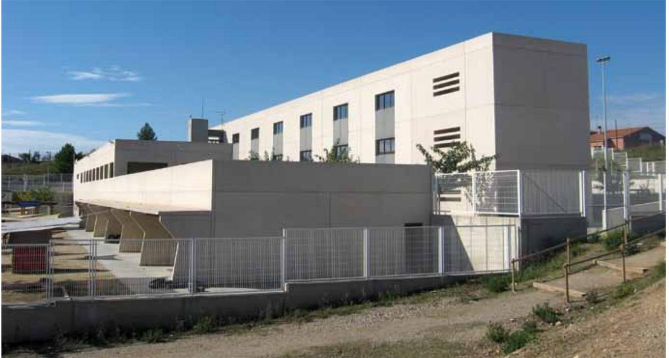
Escola Vinya del Sasret in Sant Esteve Sesrovires, Spain, was built in 2005 using precast concrete structural walls and slabs. It was designed by the architects J. A. Alonso and J. Abulí. The site is inclined, so it has a volume with different levels to minimize its environmental impact. **Courtesy of Oriol Pons.**
