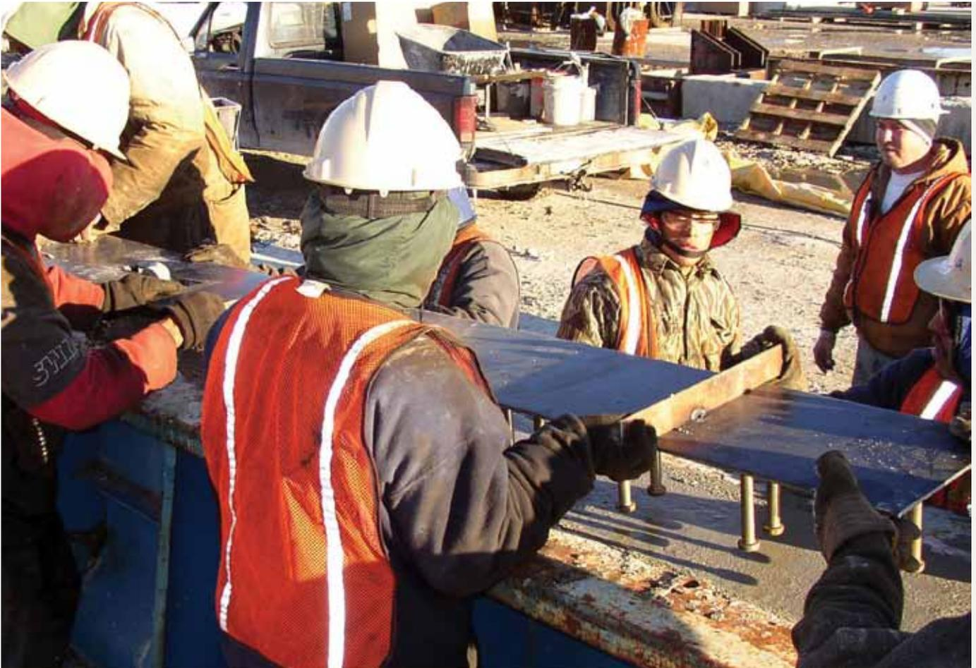
**Figure 4.** Placement of plates in girder 2.
