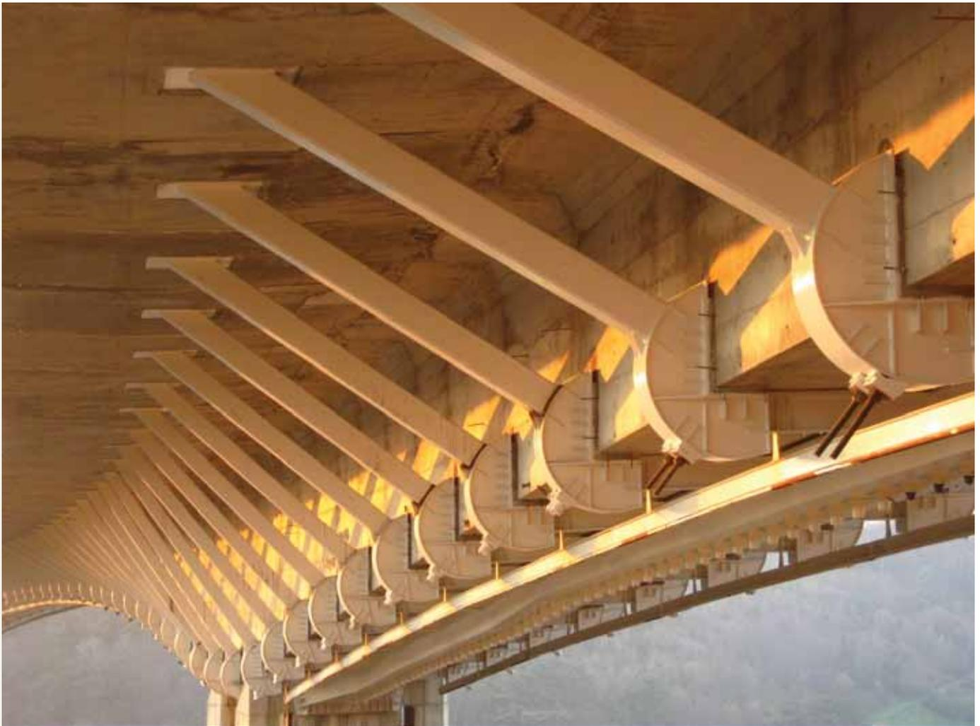
**Figure 9.** Inclined steel columns to support the cantilevers.
