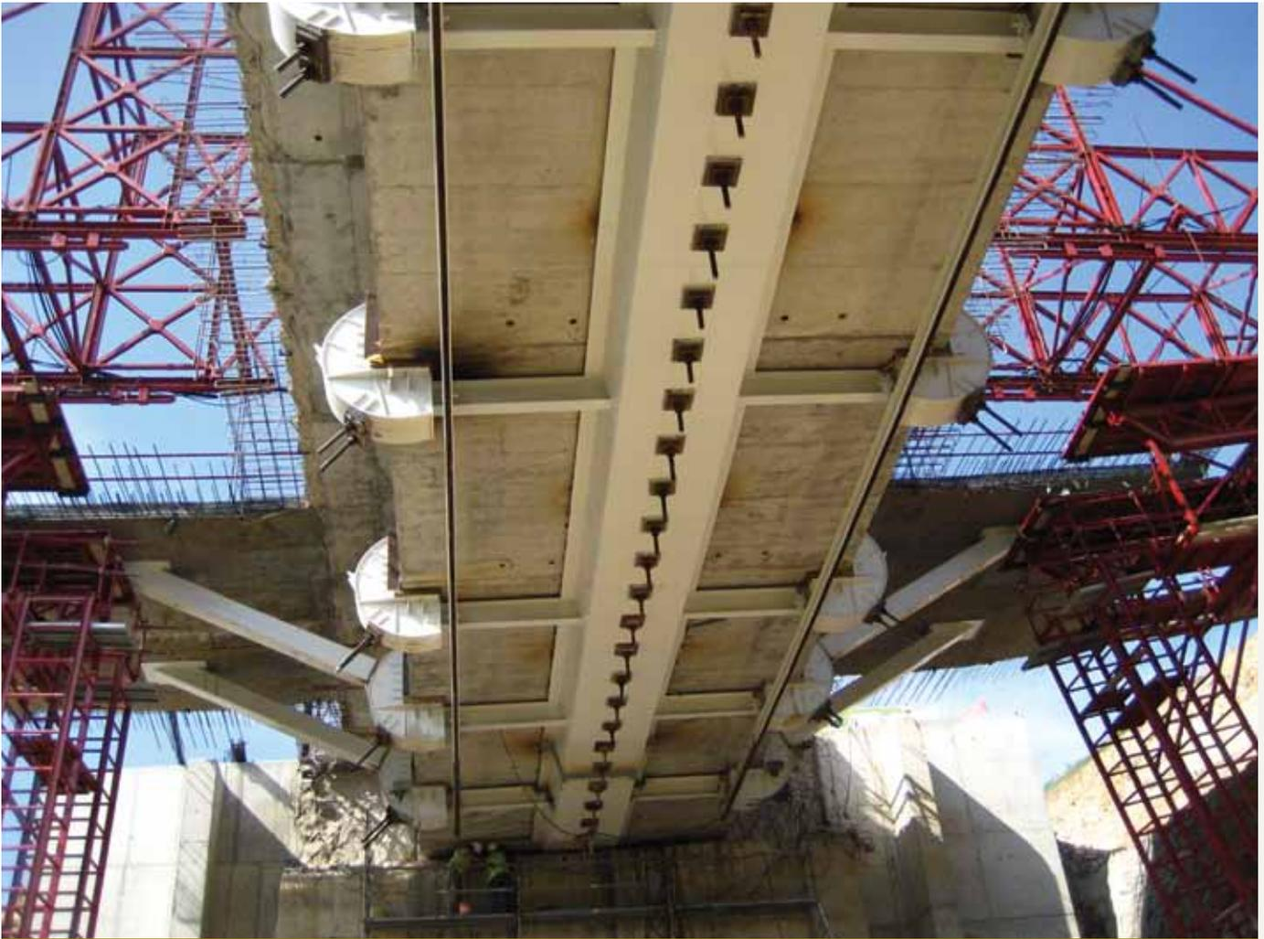
**Figure 6.** Composite box section connected to lower slab.
