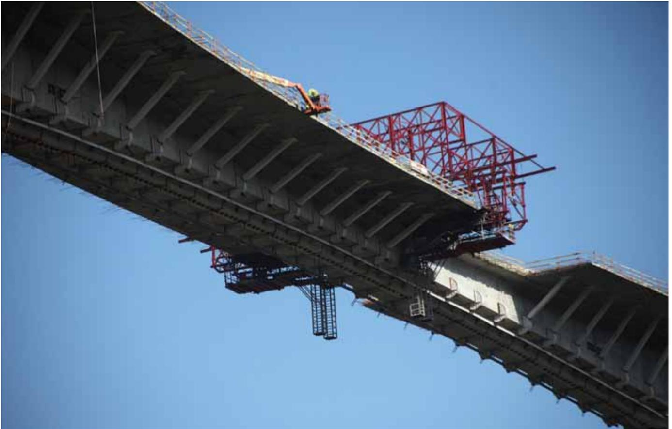
**Figure 15.** New cantilevers built with platform 3.
