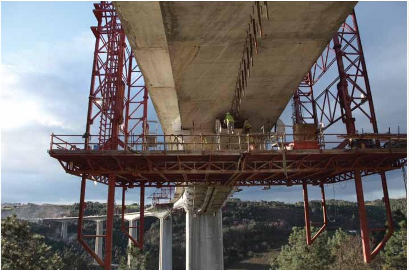
**Figure 14.** Composite box placed on-site using platform 1.
