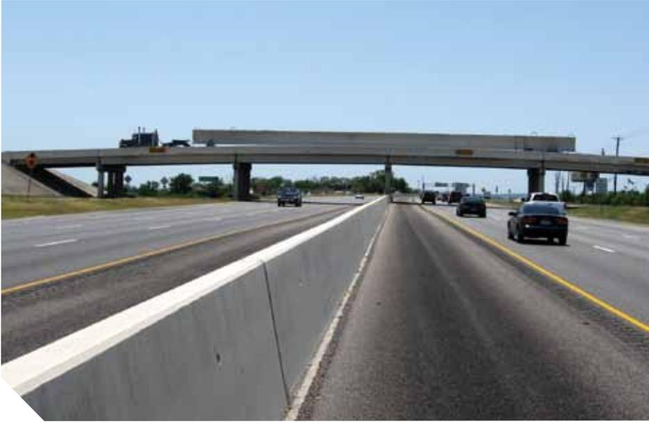
**Heldenfels Enterprises Inc. recently produced and delivered the longest prestressed concrete bridge beams ever manufactured for a Texas bridge project. Beams are being transported over an overpass to get to the jobsite. Courtesy of Heldenfels Enterprises Inc.**
