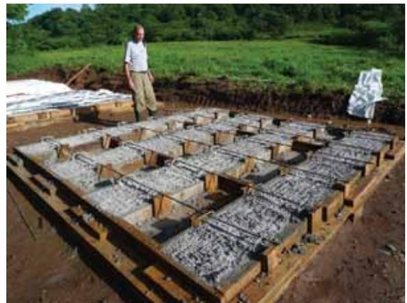
These precast concrete casting beds were used to produce match-cast deck panels for a bridge under construction by Engineers Without Borders in Canchias, Honduras. Courtesy of Dale Thomas of CH2MHill.
