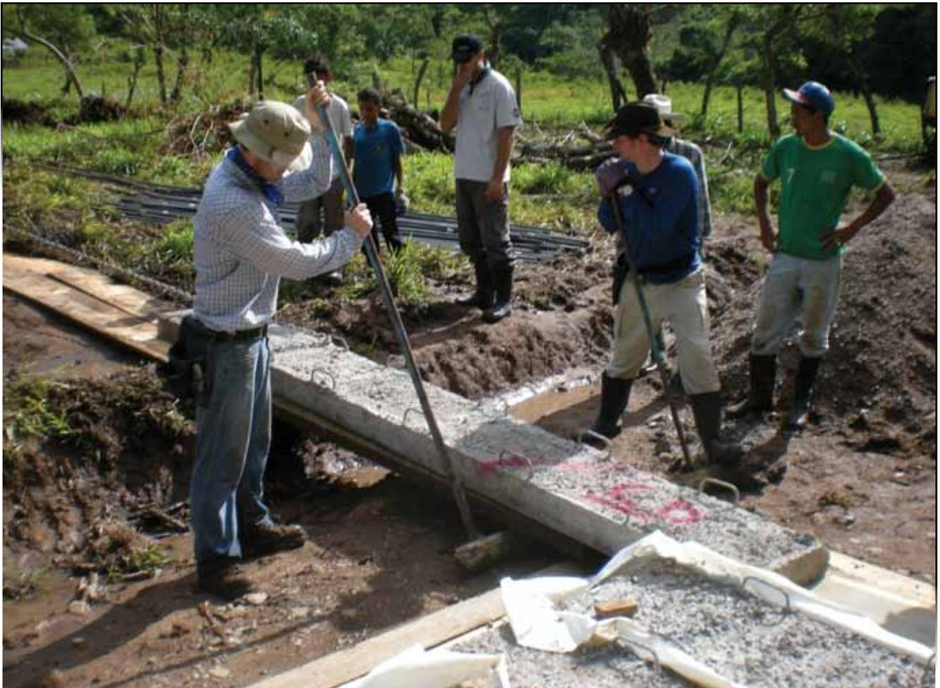
Workers with Engineers Without Borders remove the precast concrete panels from the casting bed to be stored nearby for use in a bridge in Canchias, Honduras. Courtesy of Andy Kuby of AES Due Diligence.
