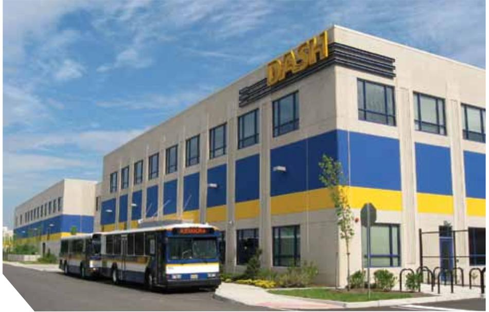
**This rendering shows the DASH William B. Hurd Maintenance Operations and Administration facility in Alexandria, Va. High Concrete Group LLC was subcontracted to fabricate insulated wall panels and precast concrete double tees for the project. Courtesy of High Concrete Group.**
