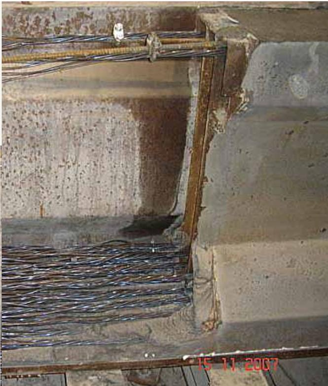
**Figure 7.** End zone of test girder B after release.
