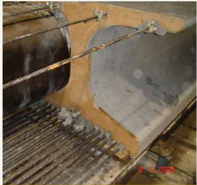
**Figure 10.** End-zone cracking in girder B.
