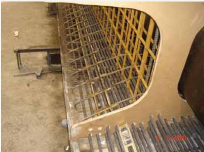
**Figure 9.** End-zone reinforcement detail of girder B.
