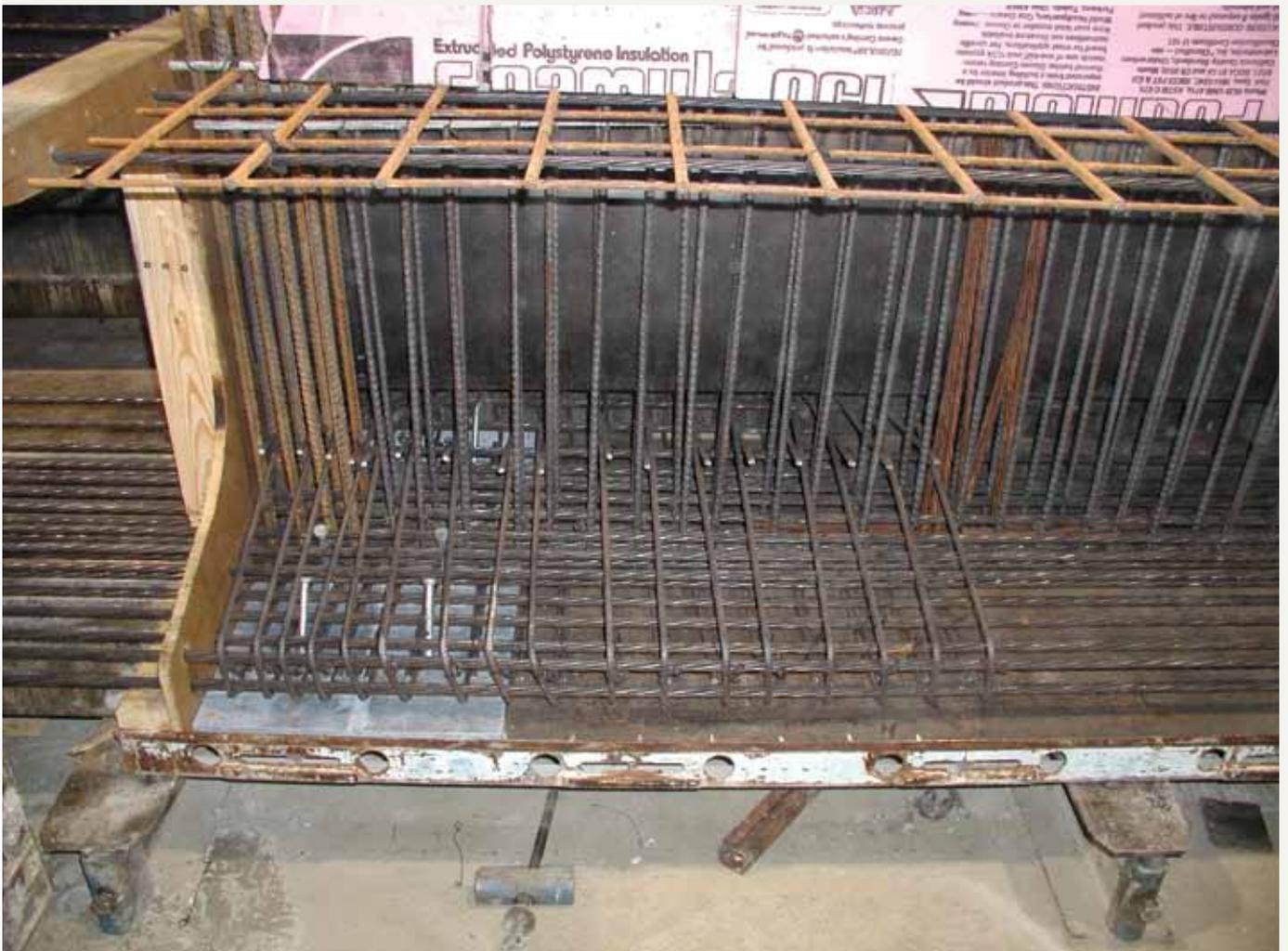
**Figure 6.** End-zone reinforcement.
