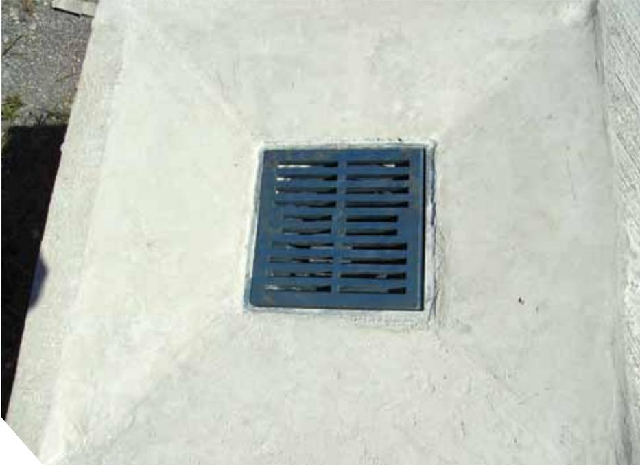
**High Concrete Group delivers double-tees with drain bodies already cast in, saving field labor.**
