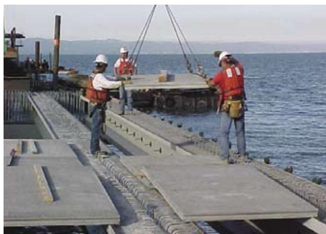
**Fig. 1.** Precast concrete slabs are being placed on precast, prestressed concrete girders for widening the San Mateo-Hayward Bridge.
