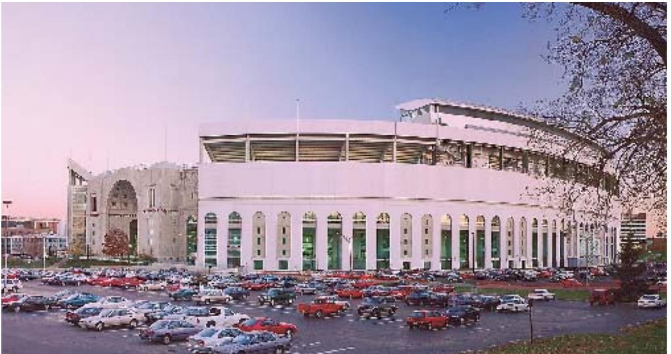
Fig. 22. The new precast exterior serves to complement, rather than compete with, the existing construction.
