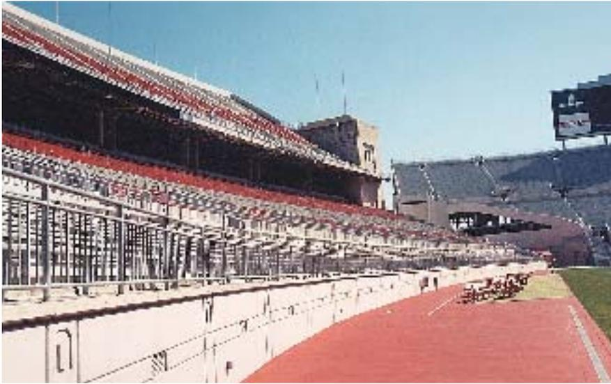
Fig. 16. Architectural precast concrete fascia walls at playing level provided owner-pleasing detailing of the OSU block “O” logo.
