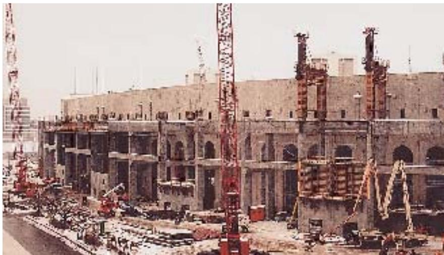
Fig. 13. Cast-in-place concrete columns and platforms provide structural support for precast expansion for the new Upper C deck.
