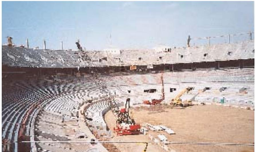
Fig. 10. New playing surface, excavated down 14 ft (4.3 m), places the playing field almost 6 ft (2 m) below the groundwater table.
