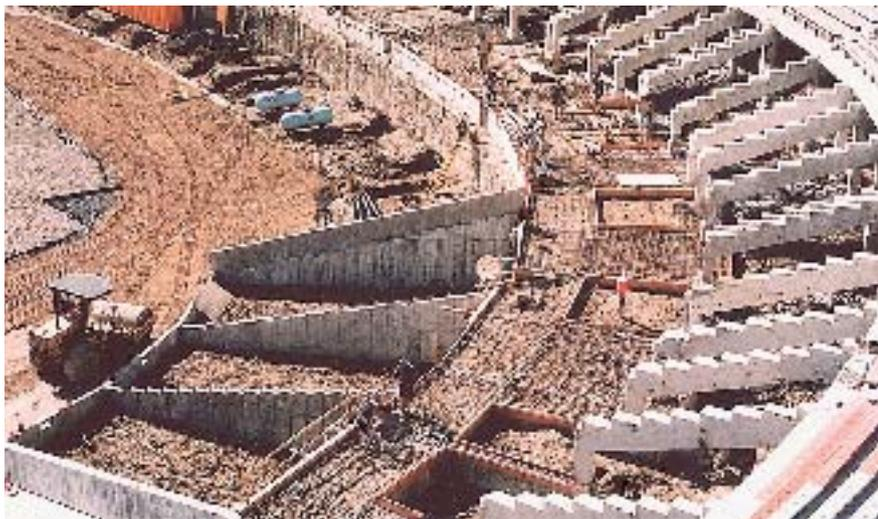
Fig. 8. Erection of the structural precast concrete raker beams at the excavated Lower AA Deck.
