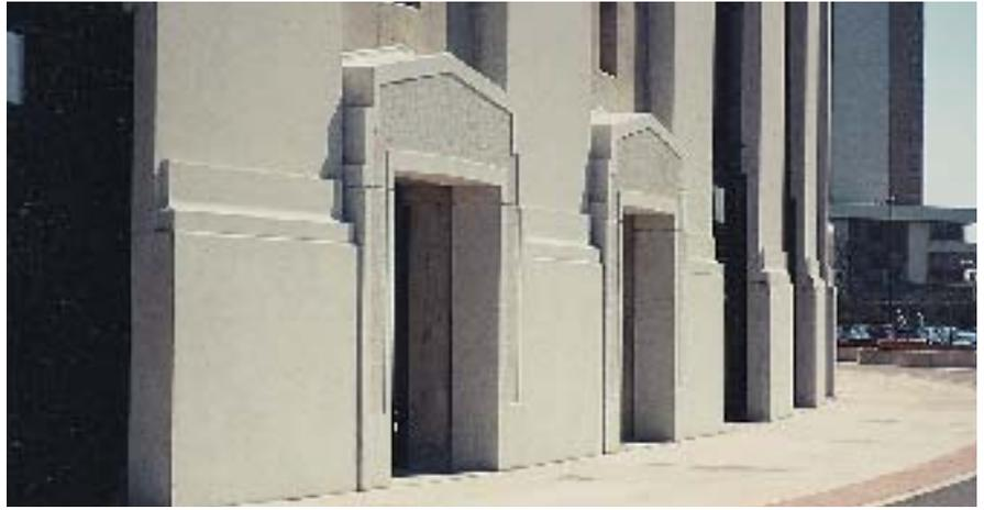
Fig. 20. Entrance portals were given a bush-hammered finish to work in aesthetic harmony with the older existing cast-in-place concrete.
