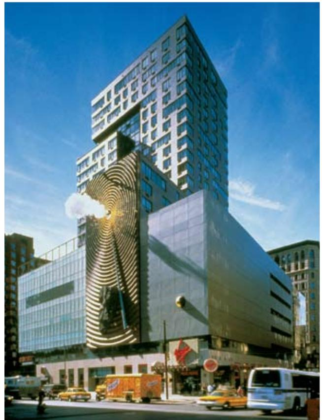
*The art wall sculpture on the Metronome building at One Union Square in New York City consists of concentric, undulating circles formed by bricks inset into shaped precast concrete panels. The art wall's theme is Time: Past, Present and Future.*
