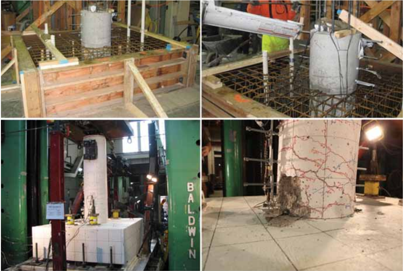
Figure 8. Construction and testing of precast concrete column-to-footing connection.
