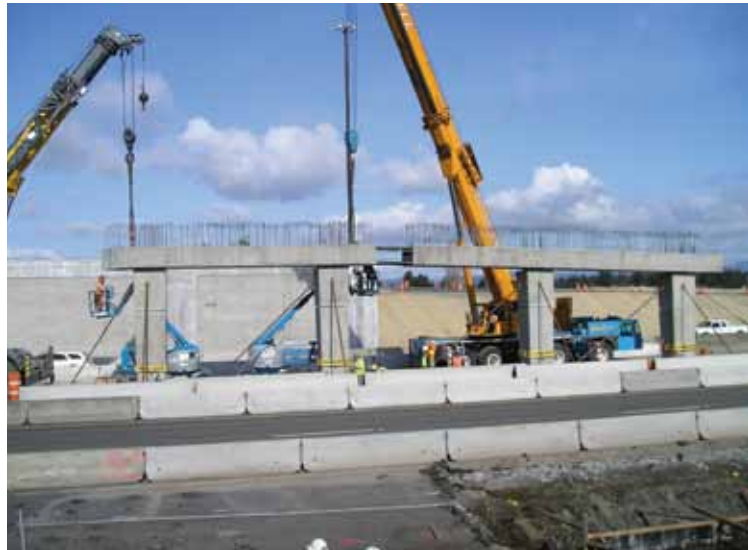
Figure 15. Placement of precast concrete cap beam.
