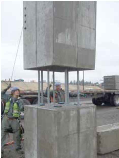
Figure 14. Placement of column segment.
