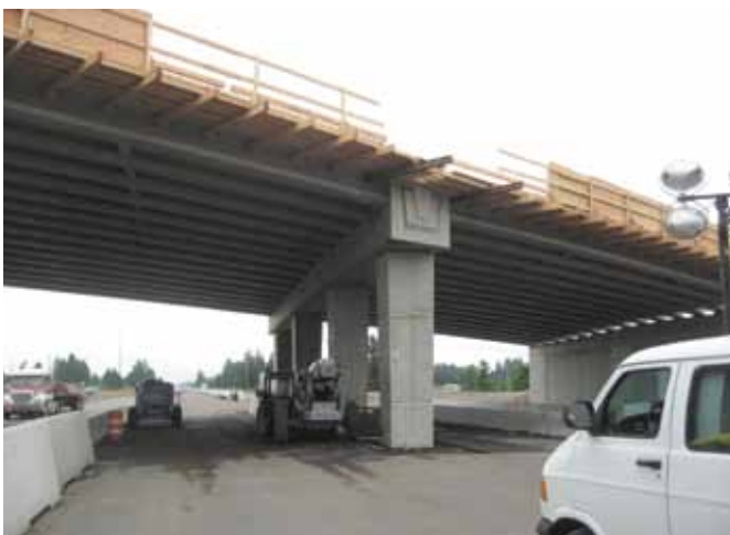
Figure 16. Placement of precast concrete girders and casting slab concrete.
