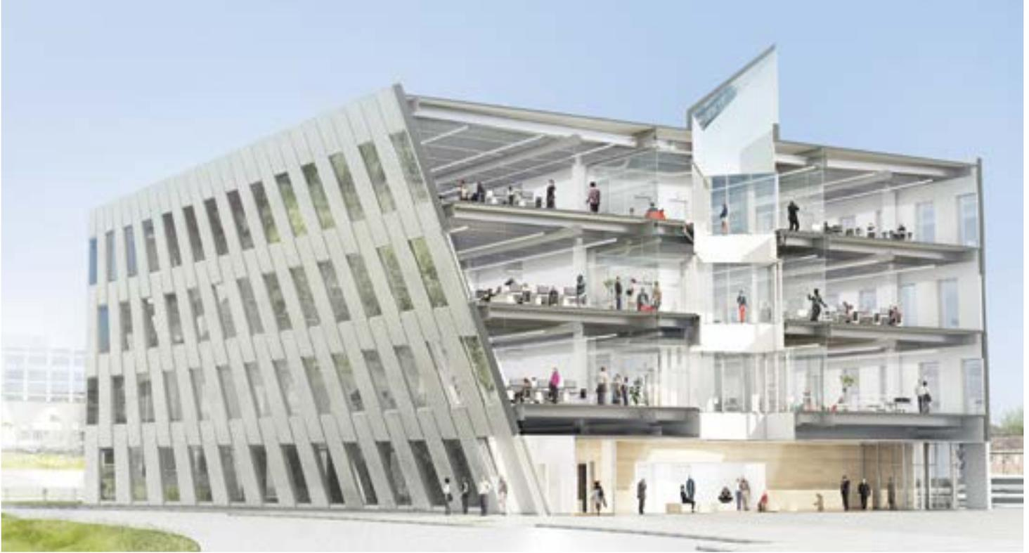
This cutaway shows how the office space adapts to the curving façade. Photo: Bjarke Ingels Group.
