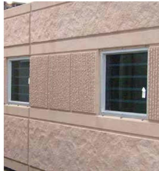
*A variety of textures were used in the architectural panels attached to the exterior of the modular cells. Photo:Tindall Corp.*
