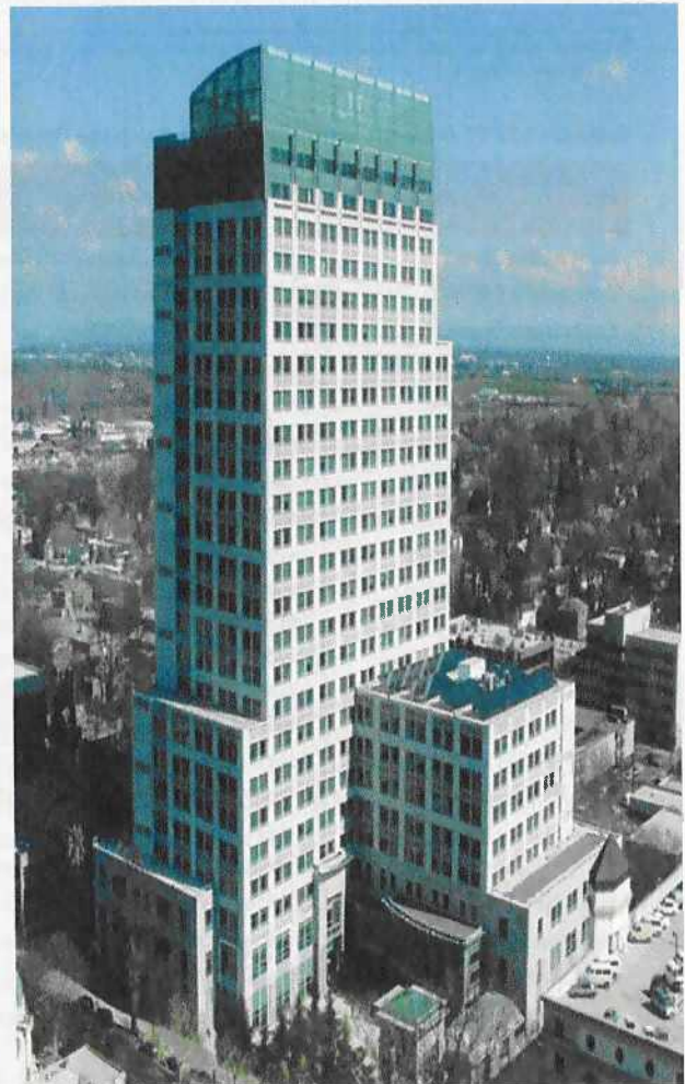
Fig. 5. First LEED Platinum certified existing high-rise. The Joe Serna Jr. California EPA Headquarters Sacramento, CA; Architect: A. C. Martin Partners.
