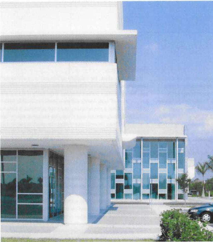
Fig. 7 High-reflecting (usually light-colored) surfaces help mitigate urban heat islands.
