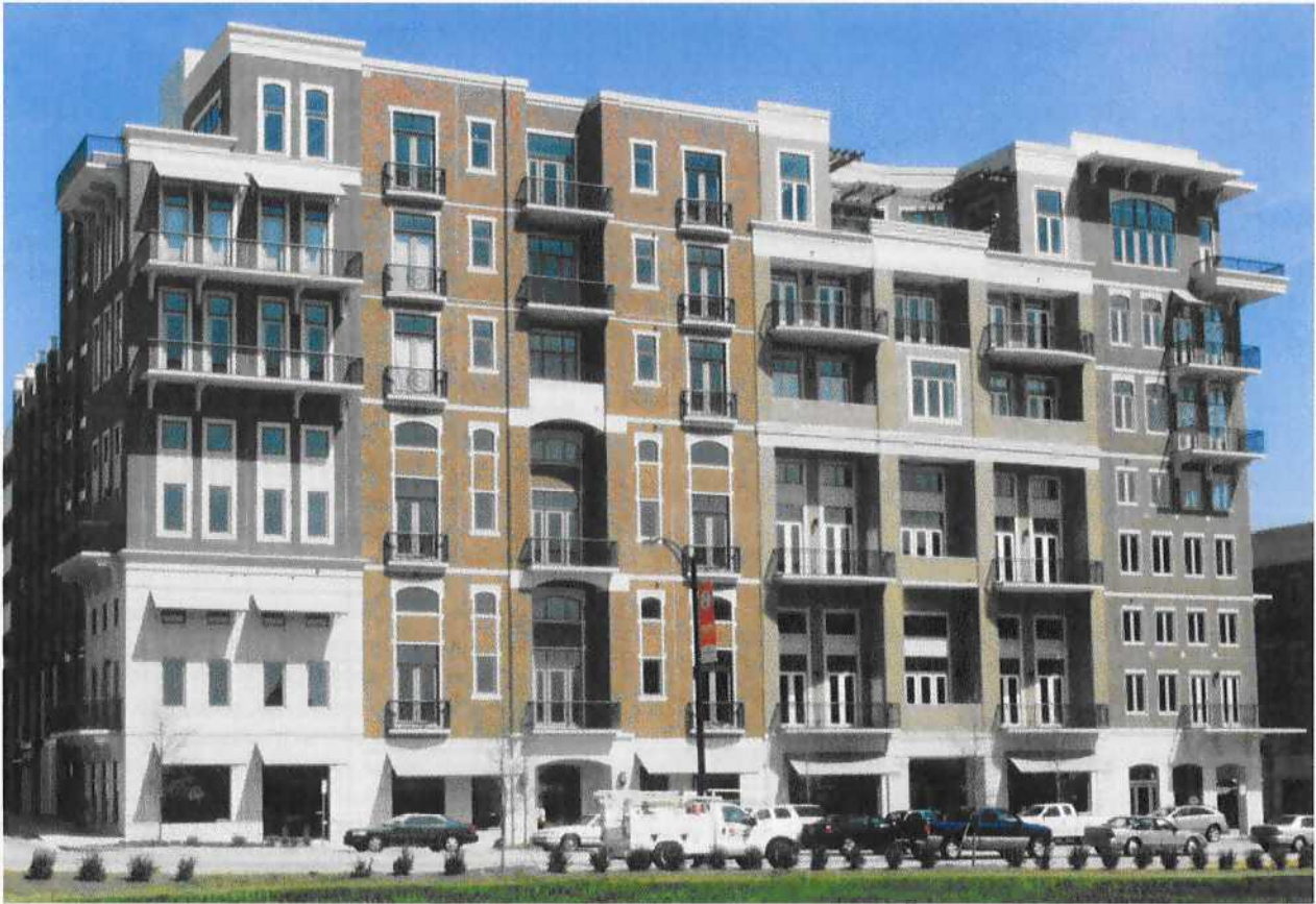
Fig. 6. LEED registered mixed-use development. Bookends, Greenville, SC; Architect & Photo: Johnston Design Group, LLC.
