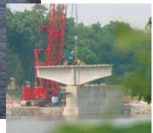
To replicate the original bridge's arched design, variable girders were cast, which required cast-in-place splices to allow them to be transported to the site safely.
