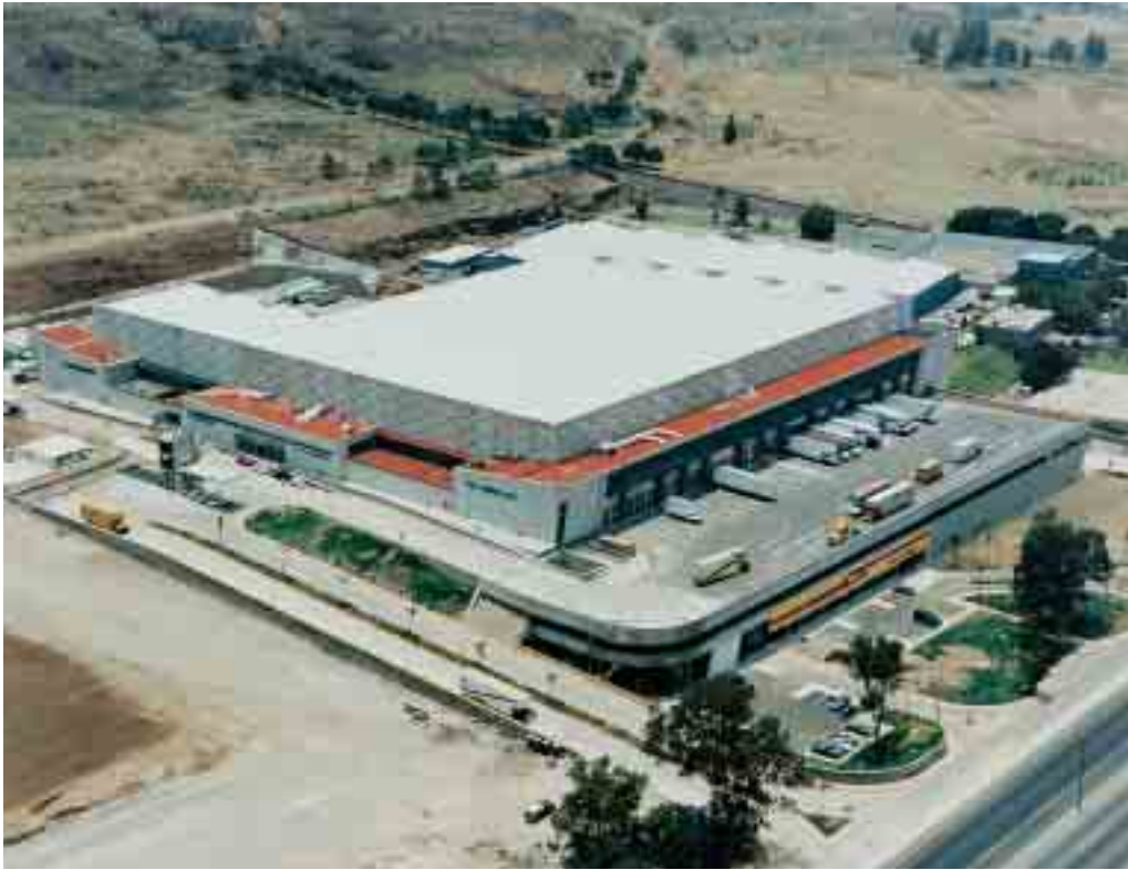
The 400,000-square-foot Elektra Guadalajara distribution center was constructed almost entirely of precast concrete.
