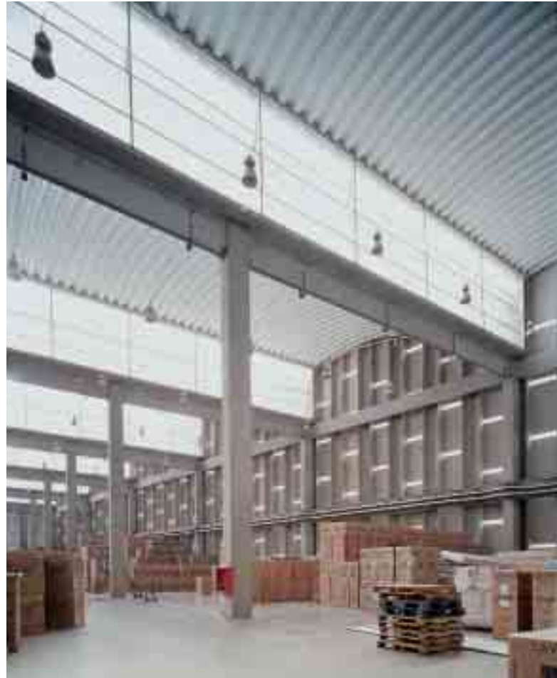
Precast columns and beams created a bright, open interior that facilitated layouts for distribution functions.
