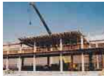
Because of the sloping site, the building was constructed with several levels. The roof of the lower level building was used as a maneuvering platform for vehicles.
