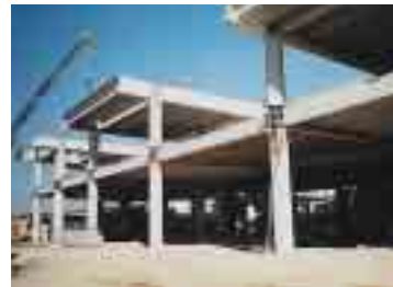
A precast concrete structure offered the most economical building material and also sped construction.
