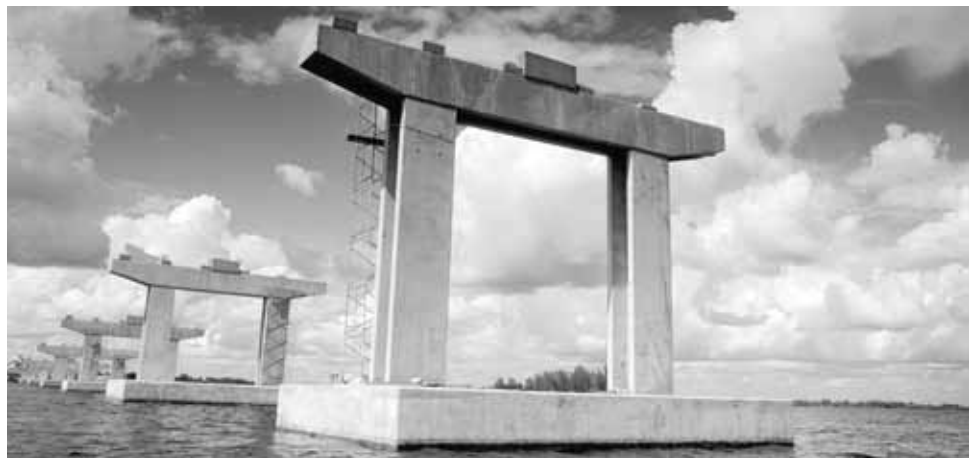
Figure 4.5.3.2-1 Edison Bridge Ft. Meyers, Fla, showing precast concrete columns and caps
