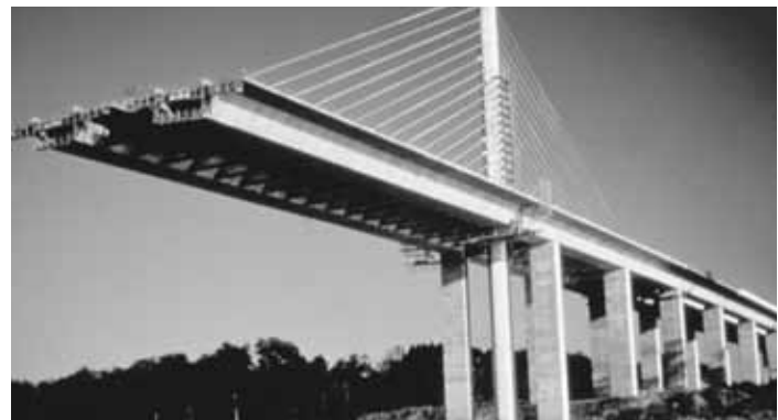
Figure 16.6-4 Finished Pier Columns, C & D Canal Bridge
