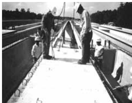
Figure 16.2.1-1 SIP Panel Erection between Precast Concrete U-Beams
