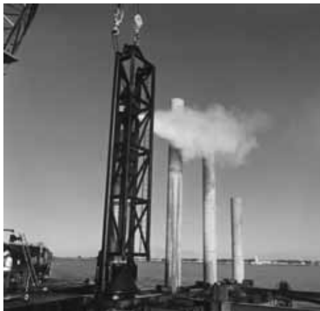
Figure 16.4.4-1 Driving Cylinder Piles
