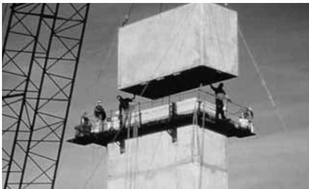
Figure 16.6-3 Erection of Pier Column Segment
