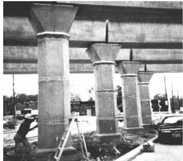
Figure 16.6-2 Columns and U-Beams at Louetta Road Overpass
