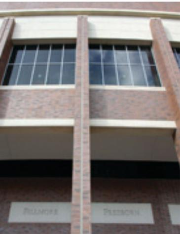
Exterior façade features thin brick inlay, precast concrete wall panels.
