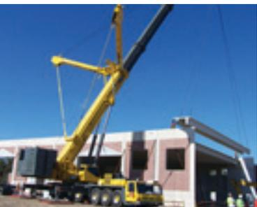
A 150-ton crane erected four precast concrete double-tees per day.
