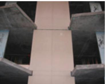
Precast panels fit snugly around balconies and other projections.
