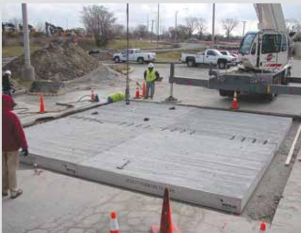
**Figure 12.** Illinois Tollway intermittent repair system. Note: 1 in. = 25.4 mm; 1 ft = 0.305 m.
