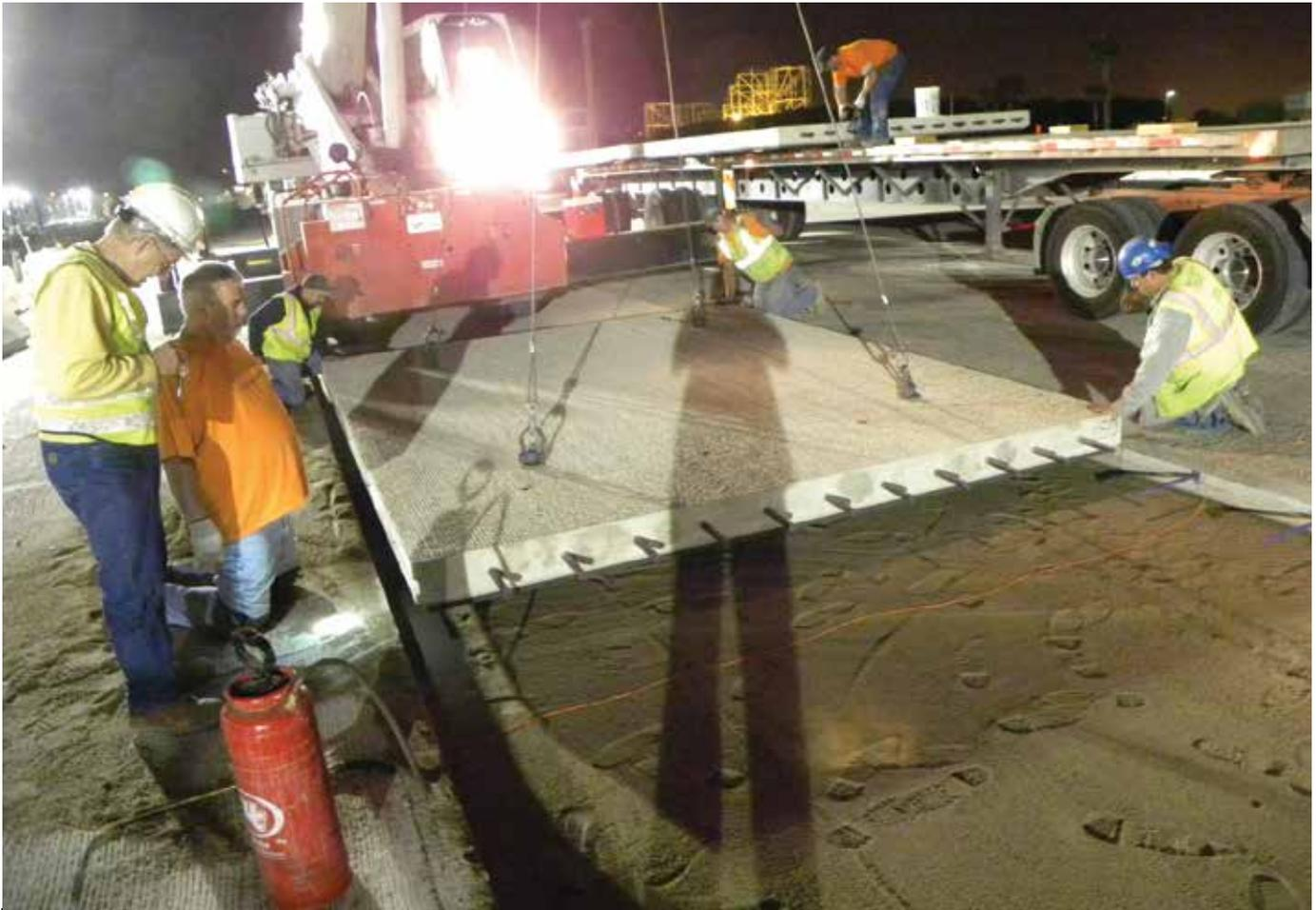
**Figure 13.** Poorly compacted fine-grained bedding layer.
