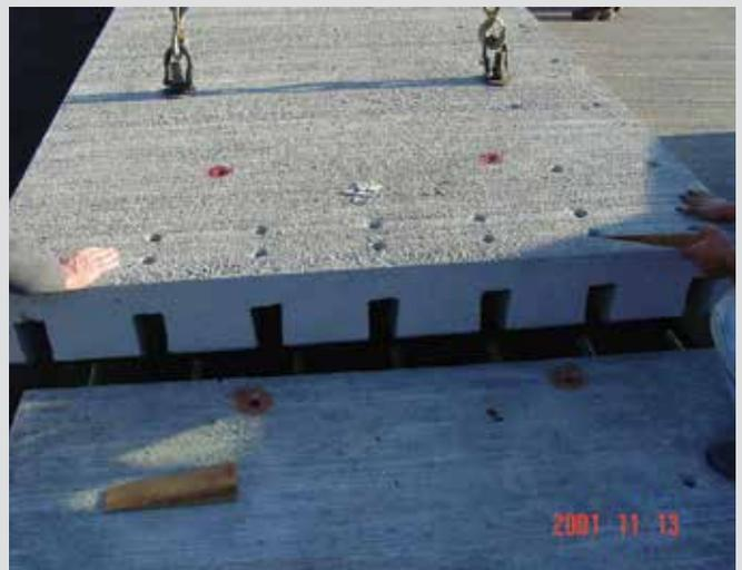
**Figure 5.** A scheme for providing load transfer in jointed precast concrete pavement.
