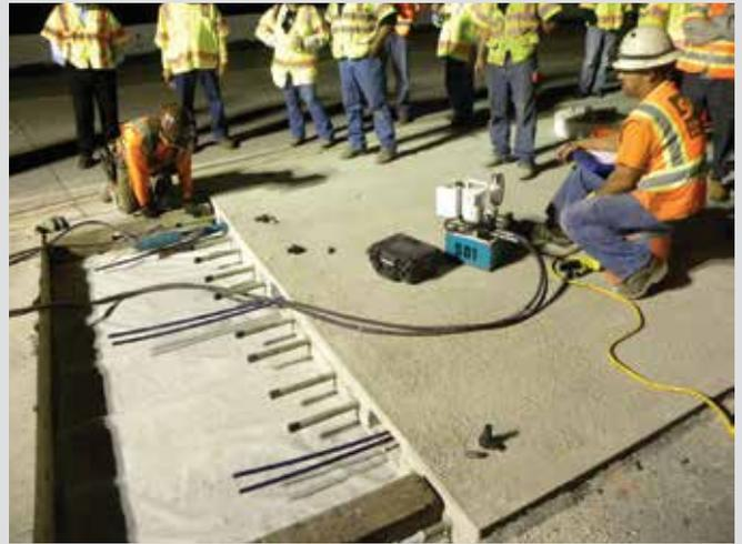
**Figure 8.** Views of the installation of two current versions of precast, prestressed concrete pavement systems.
