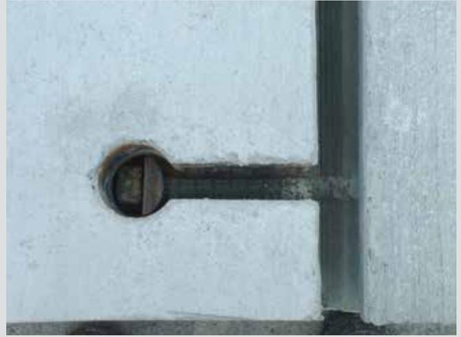
**Figure 11.** Proprietary joint interlocking slab system.
