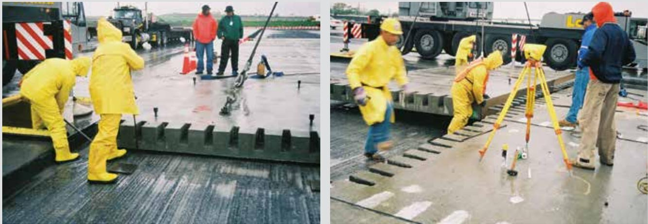
**Figure 6.** Alternative scheme for providing load transfer in jointed precast concrete pavement.
