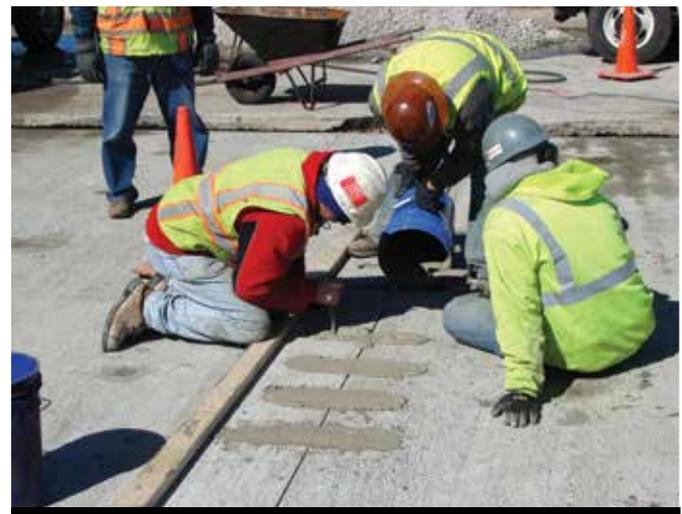
**Figure 3.** A variation for installing dowel bars using dowel bar retrofit.
