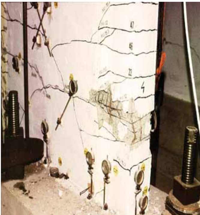
Figure 10. Precast concrete shear wall after failure.
