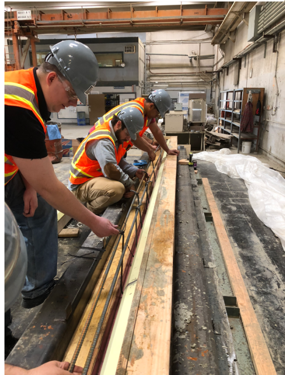
Figure 7 - Installing Reinforcement
