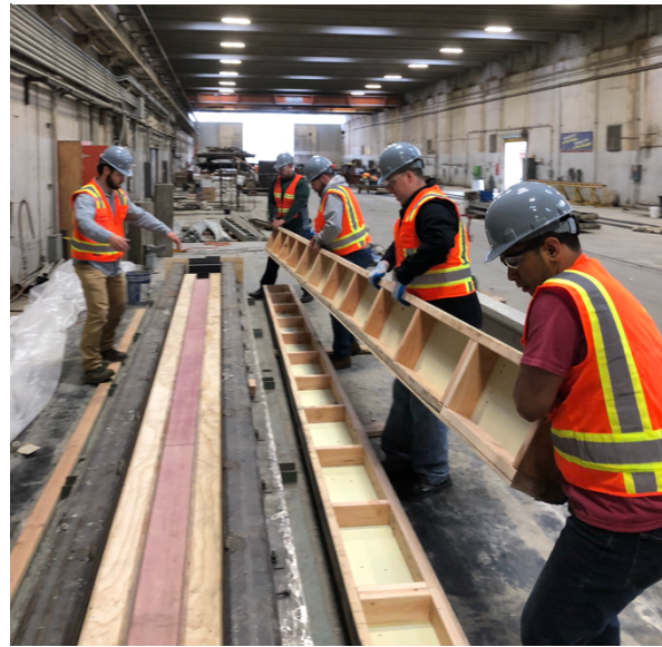
Figure 5 - Installing Formwork
