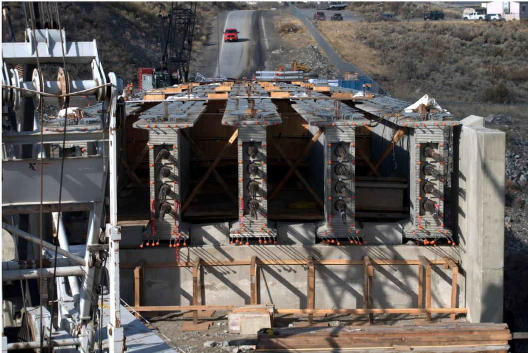
Fig. 12 Temporary Braces and Cables for Girder Stabilization
