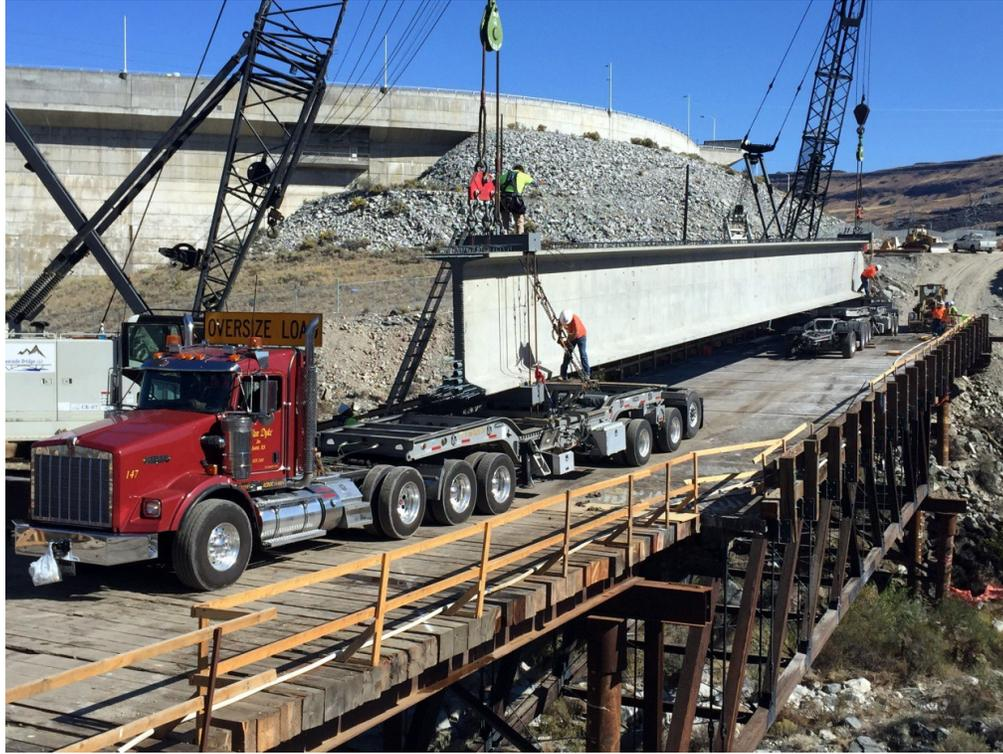
Fig. 11 Girder Installation
