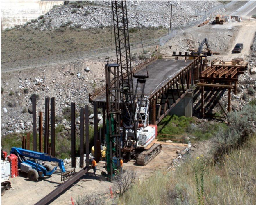
Fig. 8 Work Bridge Installation
