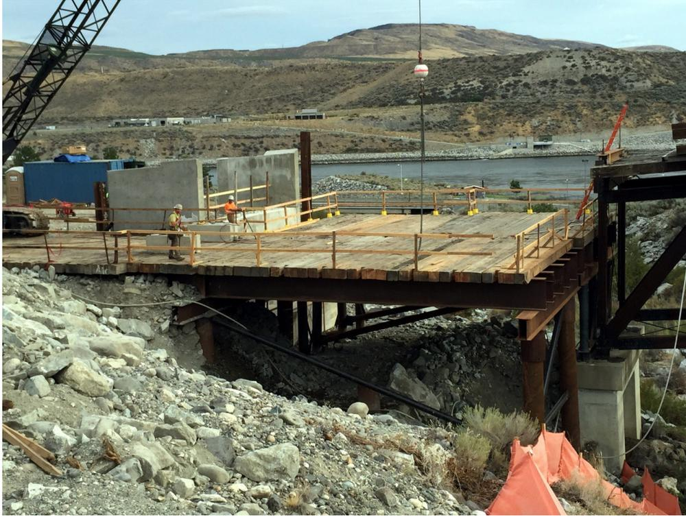
Fig. 9 Finger Work Bridge Installation
