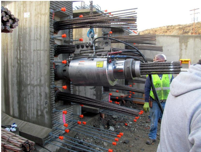
Fig. 13 Post-tensioning Application
