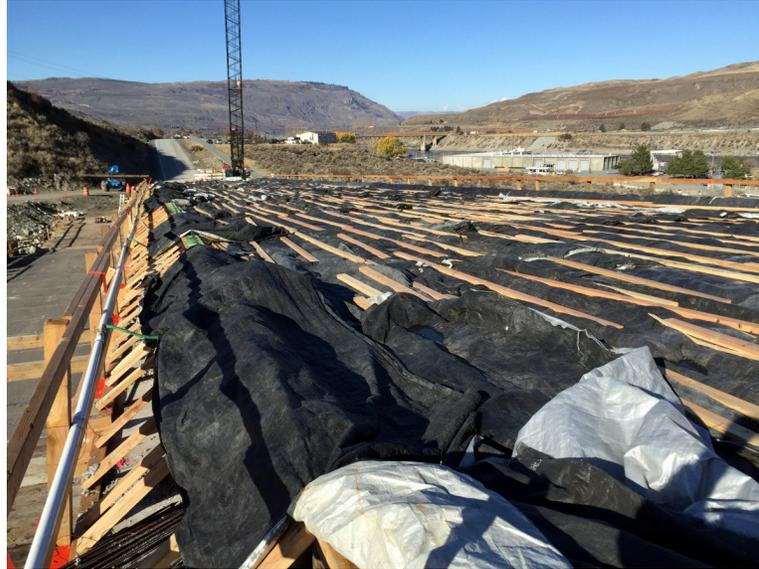
Fig. 14 Insulating Blanket on Curing Deck Concrete
