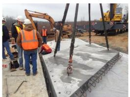
Fig. 2 Interior approach slab being set with vertical dowel alignment
