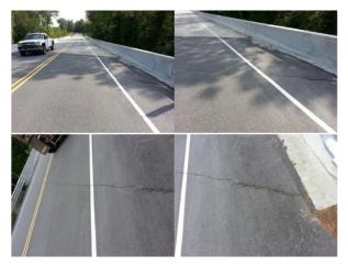
Fig.17 Photographs of observed cracks at approach slab/roadway interface (*Upper, approach to Bent Four looking south; lower, approach to Bent One looking north*)
