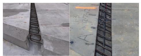
Fig. 3 Interlocking of loop bars after slab placement and (left); shear key connection joint with longitudinal reinforcing bars (right)
