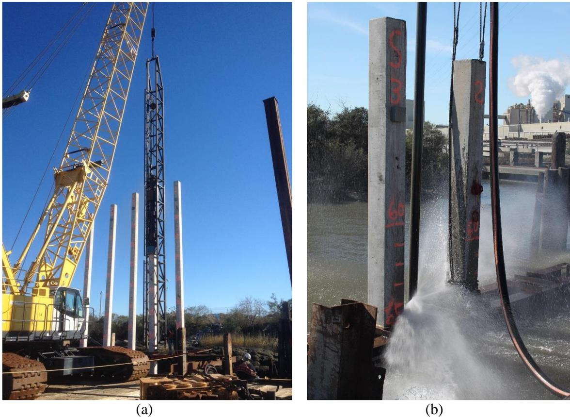
Fig. 4. (a) Driving operation of piles, (b) Extraction of piles through water jet stream applied at the bottom of the pile.
