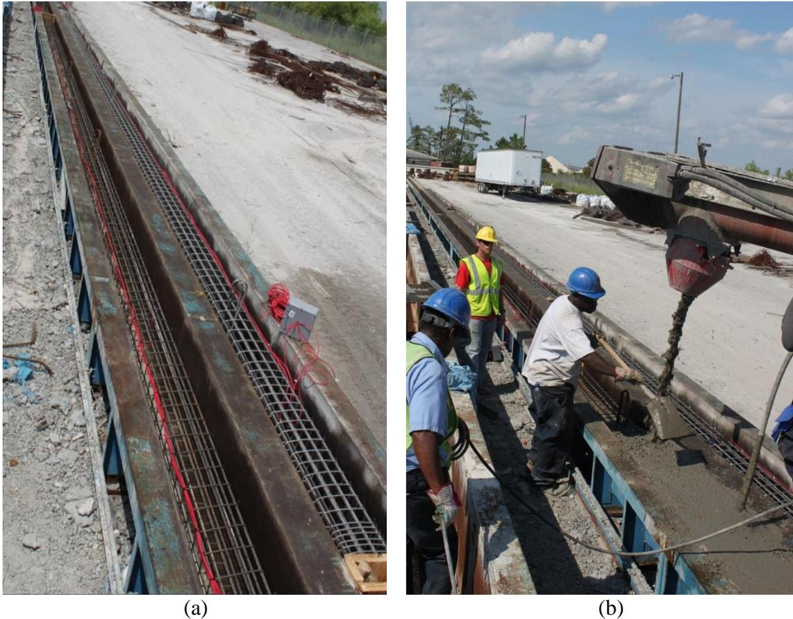
Fig. 2. Pile fabrication, (a) 1080 conventional steel strands on left, and 2205 stainless steel strands on right, (b) concrete placement operation. Piles were instrumented with vibrating wire strain gauges (red lead wire).
