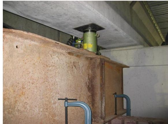
Fig. 4 Lifting from Bottom Flange
