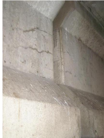
Fig. 11 Typical Anchorage Zone Cracking
