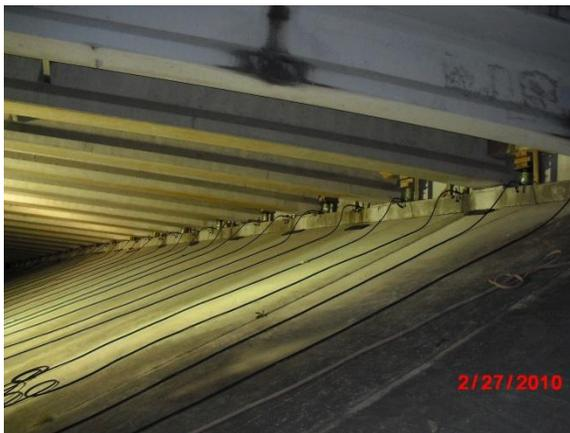
Fig. 7 Lifting from Beam Top Flange
