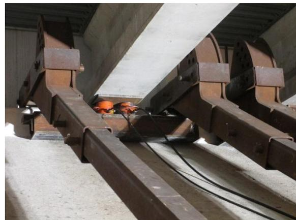
Fig. 6 Lifting from Bottom Flange
