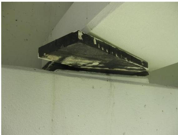
Fig. 1 Elastomeric Bearing Walk-Out
