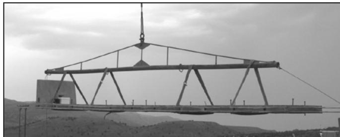
Figure 8. Third and last lift at the bridge including parapet
