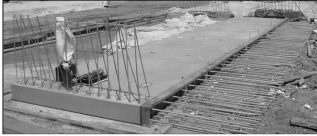
Figure 4. Panel EP3 at the precast yard with approach slab reinforcement on the right.
