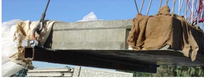
Figure 6. Panel lifting using HSS 4x4 steel tubing attached to 1" diameter steel cables.
