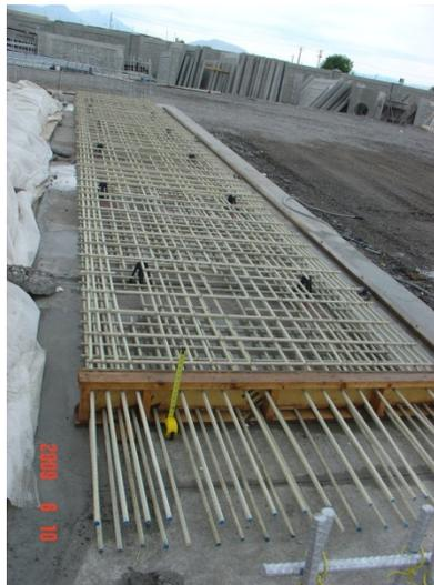
Figure 3: GFRP bar layout with bars extended for the closure pour
