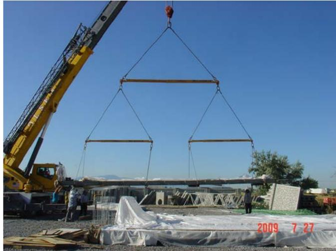
Figure 7. First lift out of the forms at the casting yard
