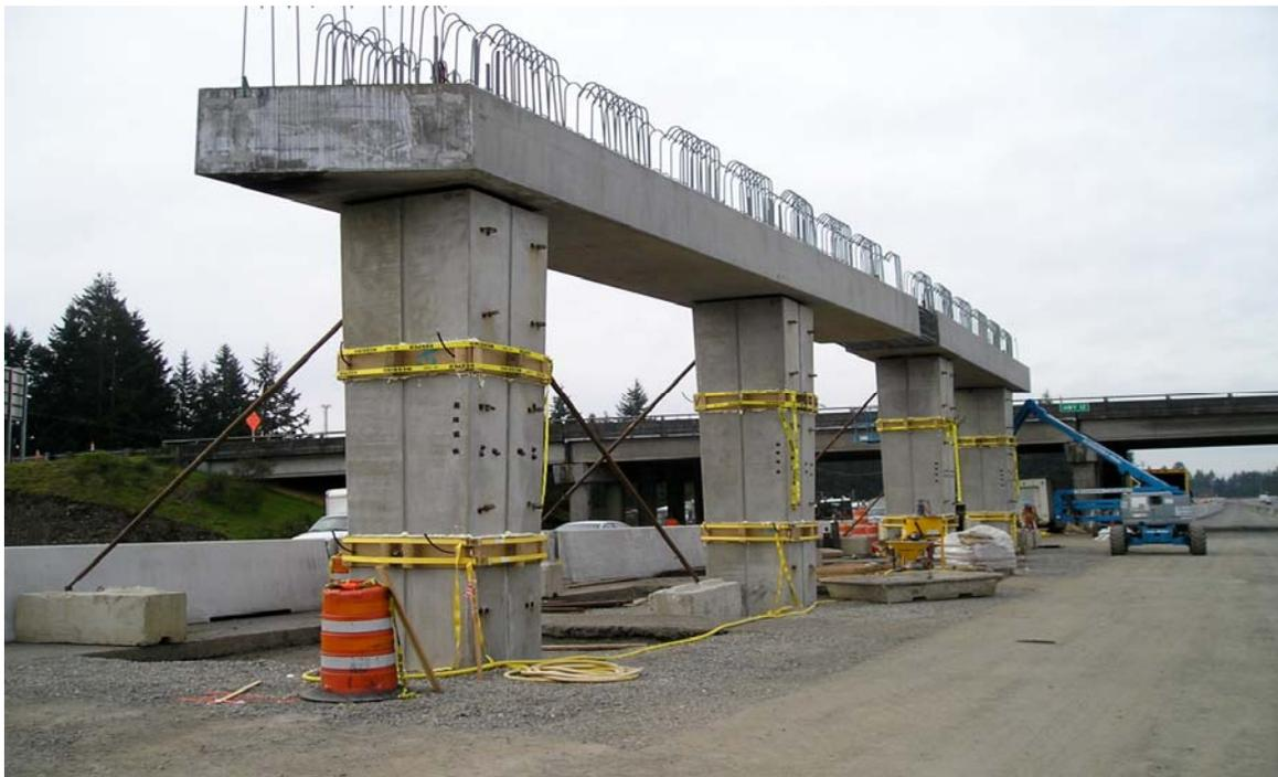
Figure 13: Grouting the Joints between Column Segments and the Column to Bent Cap
