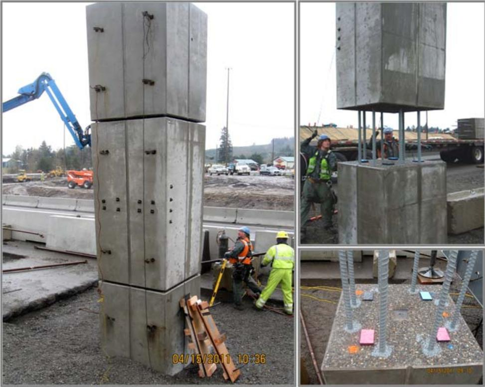
Figure 11: Column Segment Placement
