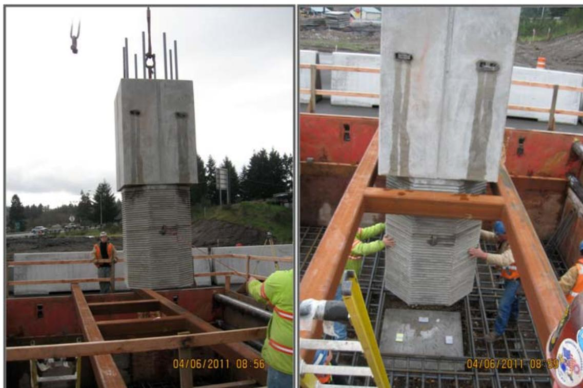
Figure 10: Construction sequences for placement of precast column segment into footing
