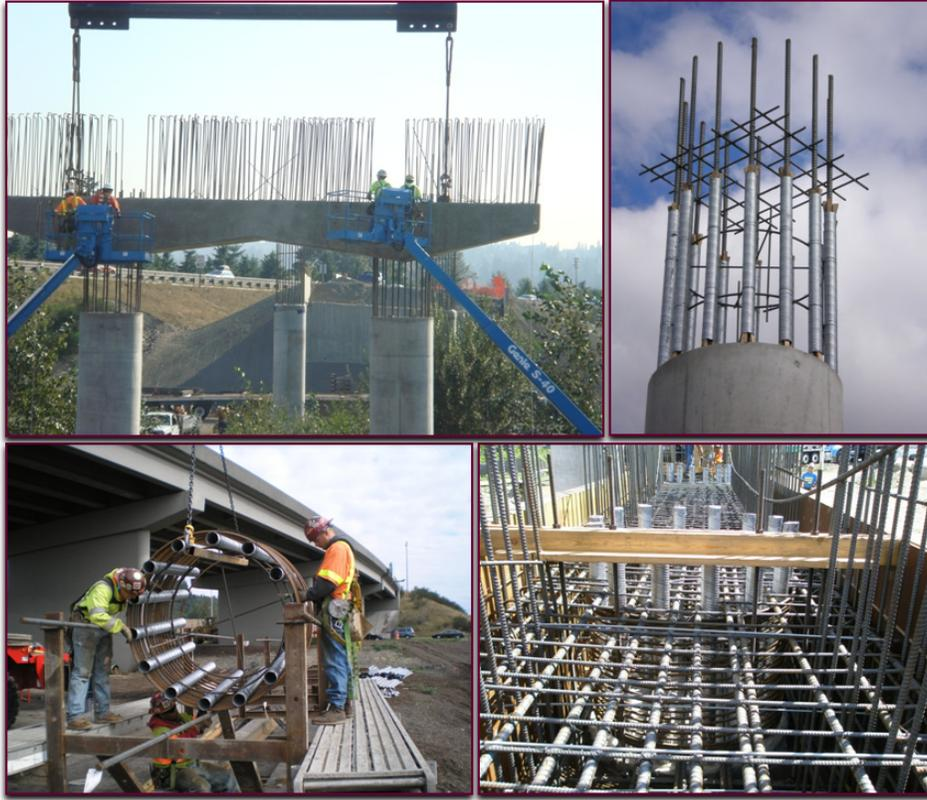
Figure 4: Precast Bent Cap under Construction in Washington State
