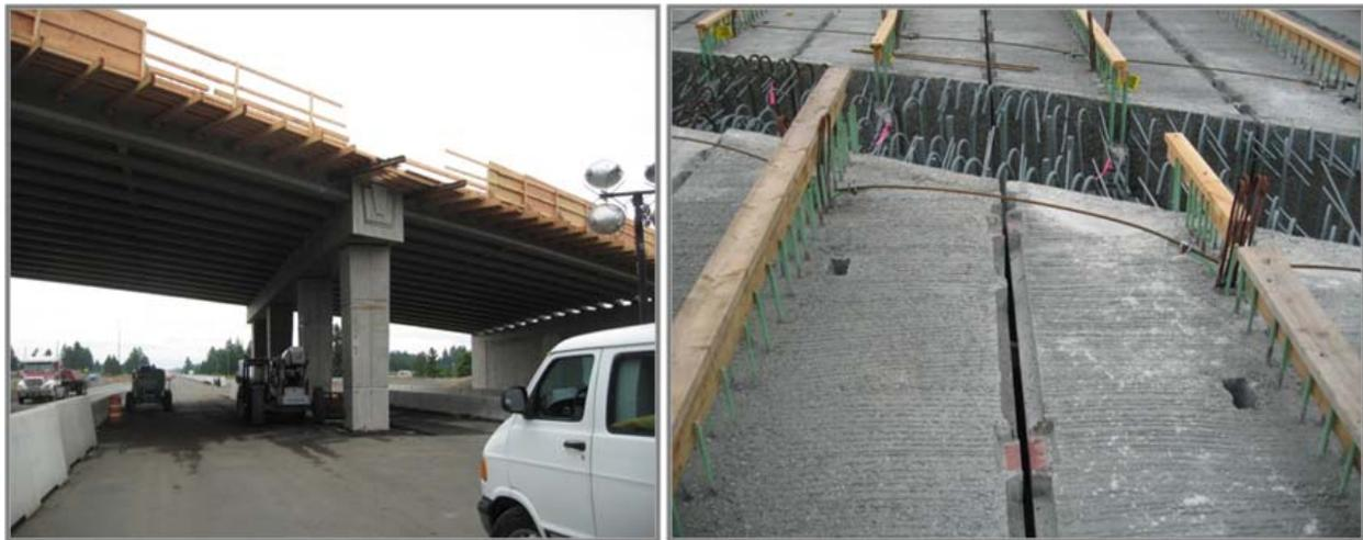
Figure 14: Placement of Precast Girders and Casting Slab Concrete
