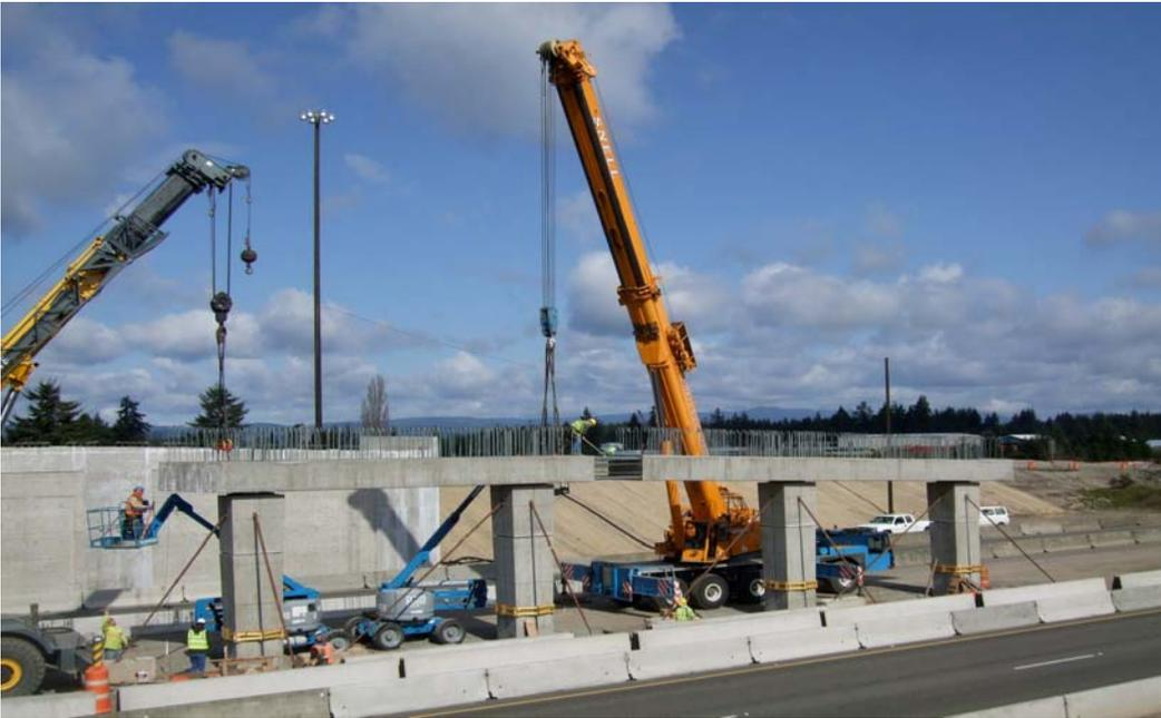
Figure 12: Precast Bent Cap Placement
