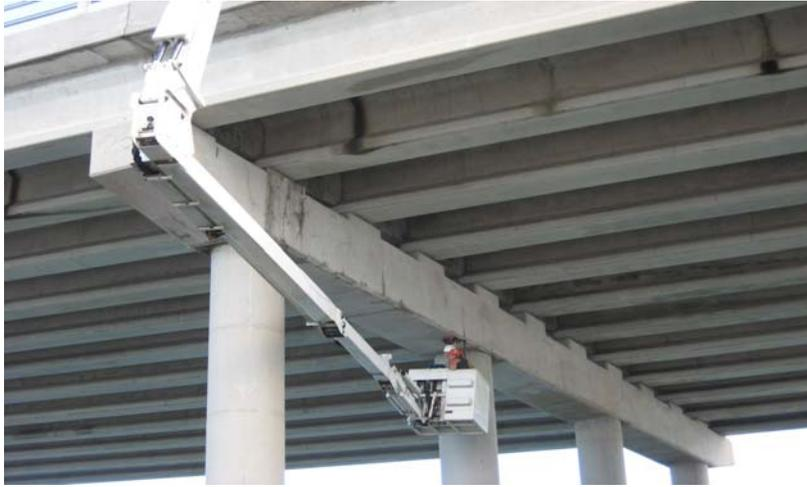
Photo 3. GPR Scan of Representative Pier Cap
