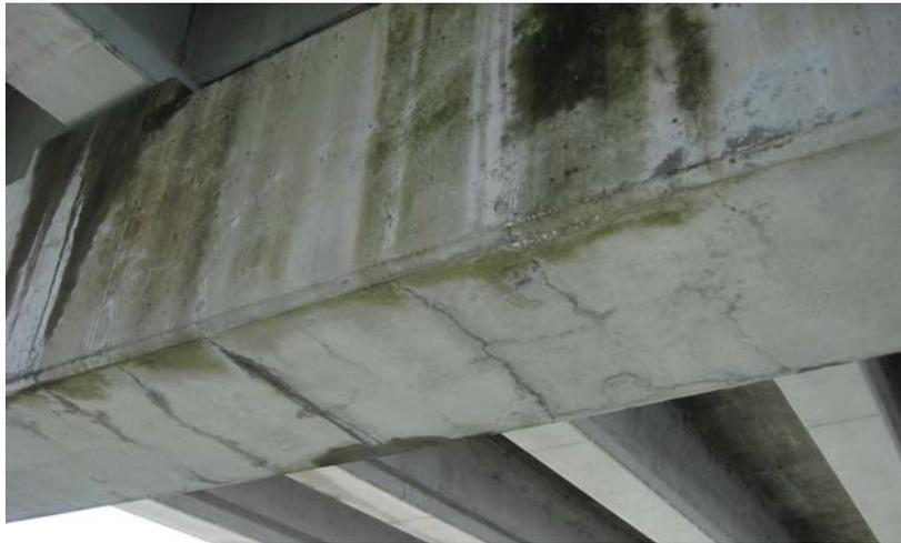
Photo 4. Typical Cracks in Positive Moment Region Between Columns
