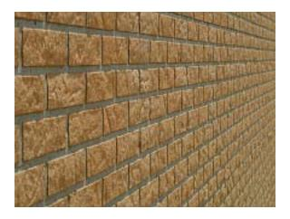
Fig. 18. Stencil-finished precast concrete panel texture
