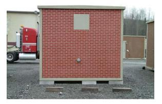
Fig. 21. Example of a communications building utilizing stencil-finished precast concrete panels
