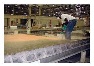
Fig. 11. Color hardener is broadcast onto concrete
