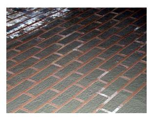
Fig. 10. Stencils are embedded flush with the concrete surface
