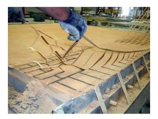
Fig. 15. Checking stencil release before removal
