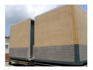
Fig. 17. Completed stencil-finished precast concrete panels
