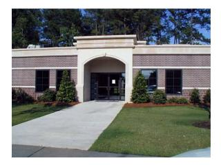
Fig. 19. Example project utilizing stencilfinished precast concrete panels
