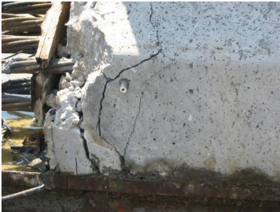
Figure 1. Bearing zone cracking due to sliding friction after strand cut-down.
