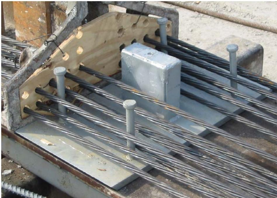
Figure 4. Galvanized embedded steel plate on prestressing bed.
