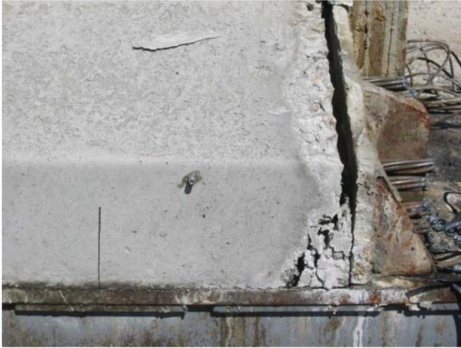
Figure 8. Cracking in Teflon Pad-2, typical
