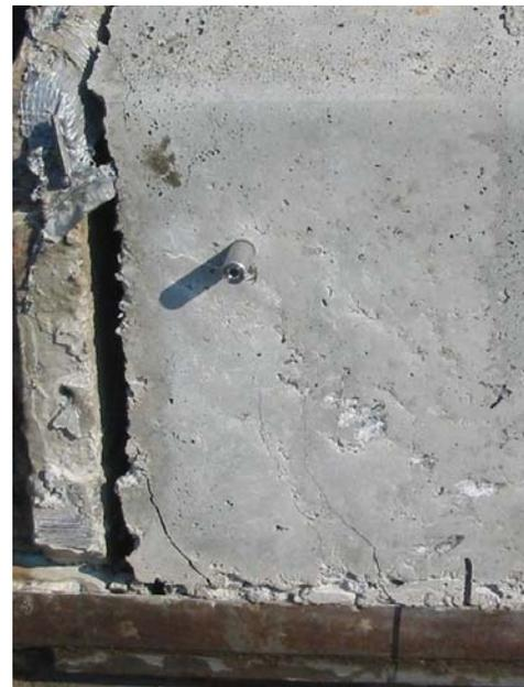
Figure 10. Cracking at one location in Angle-1 girder
