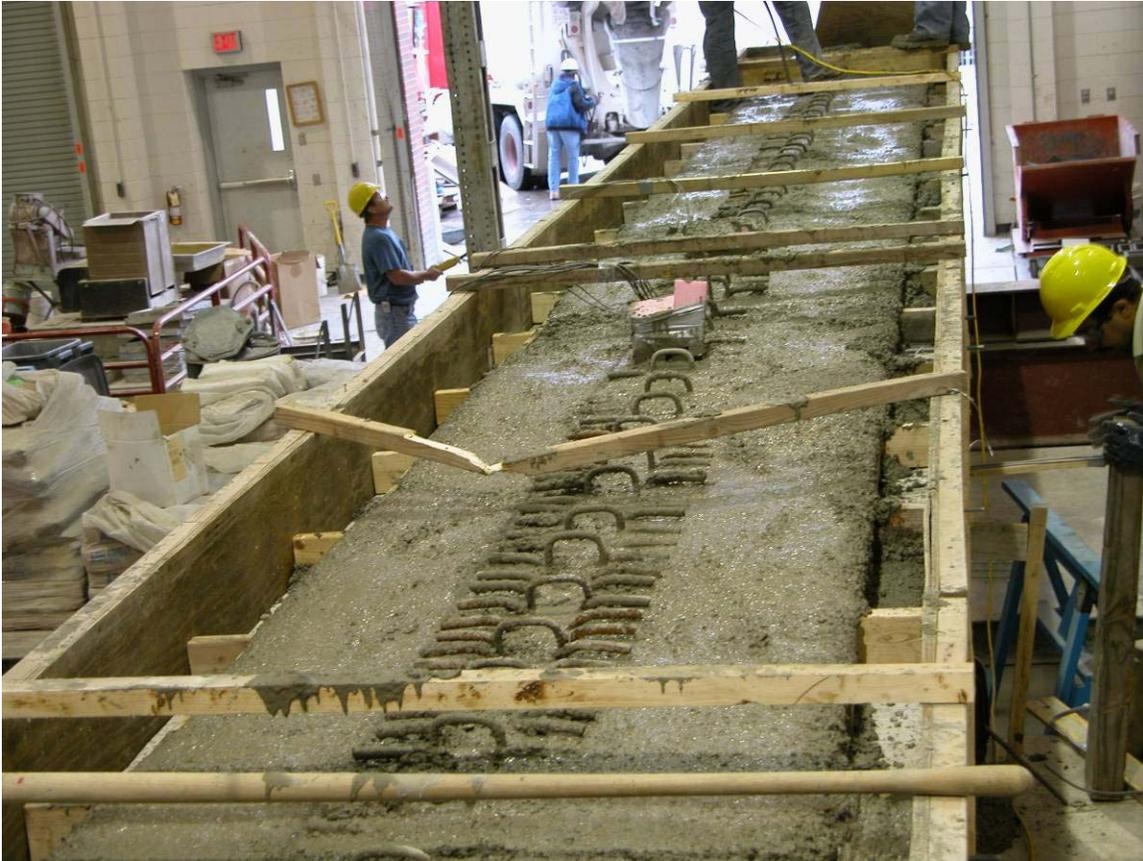
Fig. 14 Pouring Concrete Around TRs
