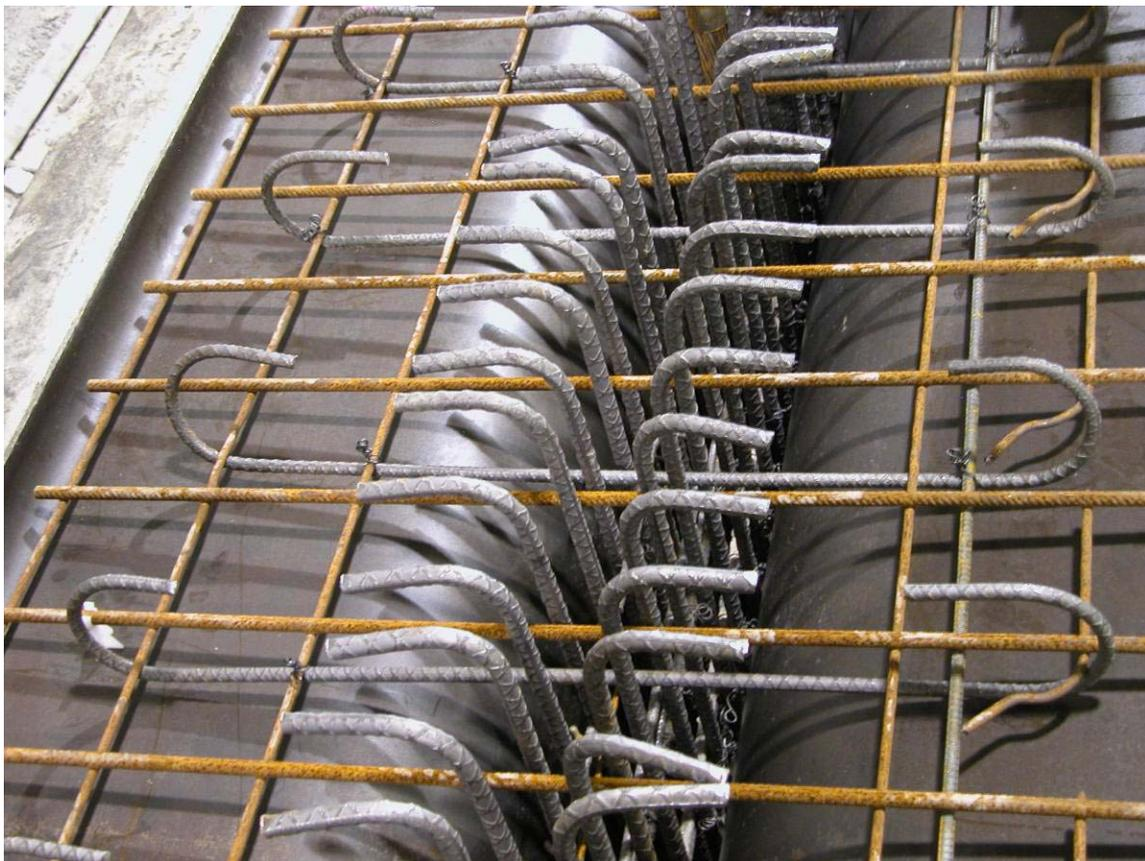
Fig. 12 C Shape Confinement Reinforcement in the Top Flange
