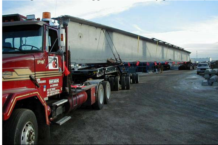
Fig. 9 Shipping a 211 ft-long girder in Bow River Bridge
