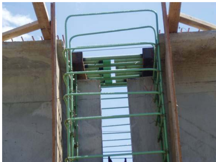
Fig. 17 Threaded Rod Continuity Details over the Pier
