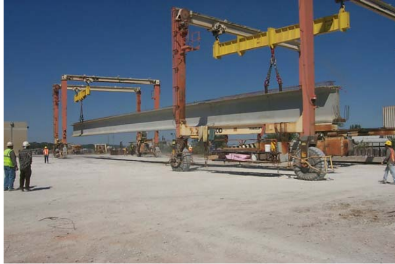
Fig. 13 Girder Handling in the Precast Yard
