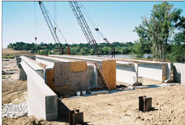
Fig. 16 (c) Girder Installation
