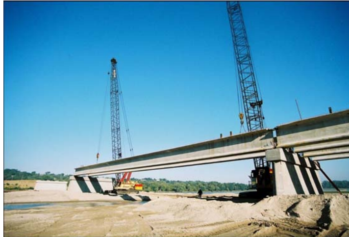
Fig. 16 (b) Girder Installation
