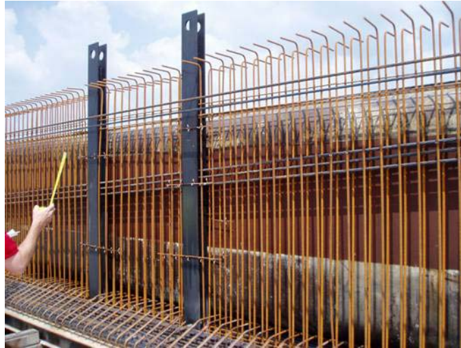
Fig. 11 (a) Girder Lifting Device Elevation
