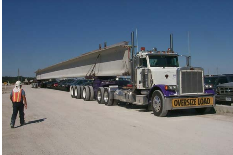
Fig. 15 Girder Shipping to the Bridge Site
