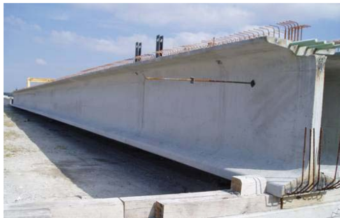
Fig. 12 Girder Stored in the Precast Yard
