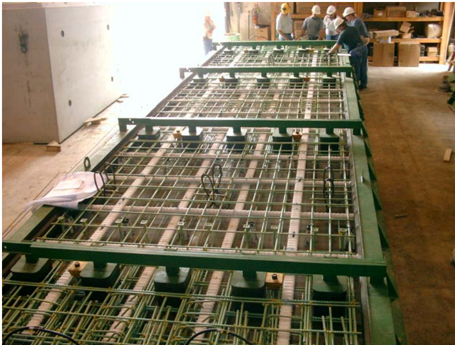
Figure 4 Typical Panel Before Casting
