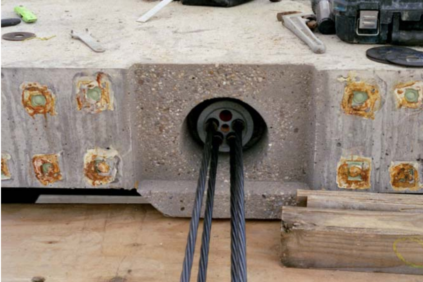
Figure 5 Typical Longitudinal Post-Tensioning Duct
