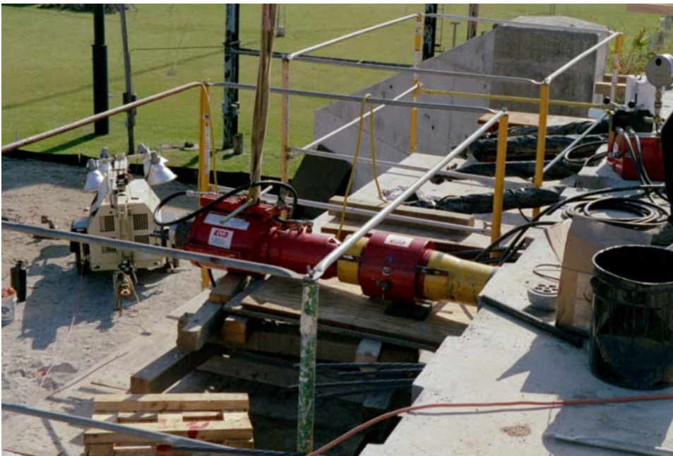
Figure 9 Post Tensioning at the Forward Abutment
