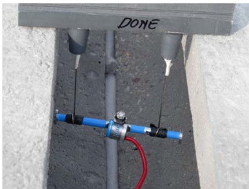
Figure 10 Vibrating Wire Gauge Placed in the Joint
