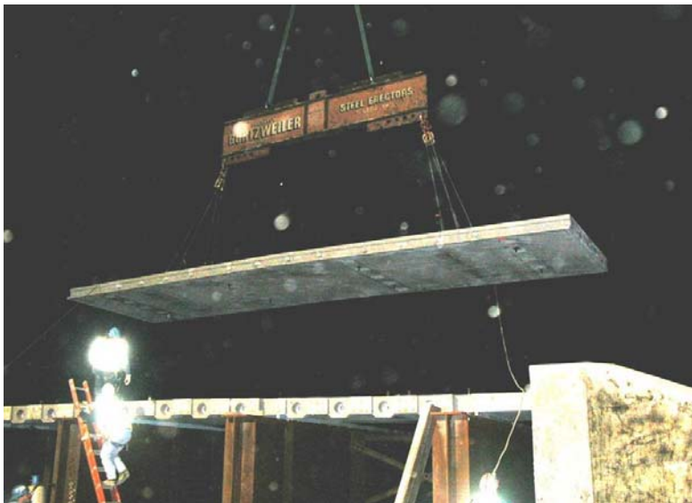
Figure 7 Placing the Precast Panels on the Steel Plate Girders
