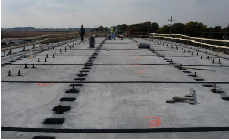
Figure 8 Top of Bridge After the Panel Placement Before Grouting the Joints
