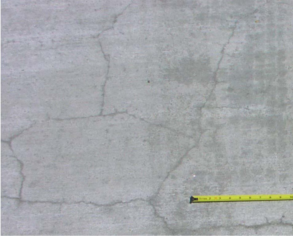
Fig. 16 Shrinkage Cracks in Overlay
