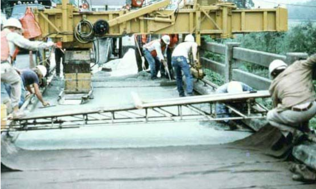
Fig. 15 Wet Burlap is Placed on the Overlay as Soon as Practical to Prevent Plastic Shrinkage Cracking
