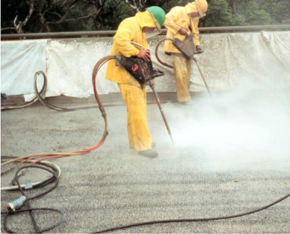
Fig. 11 Hydro Blasting Equipment Removes Approximately 1/8-in of the Deck Surface
