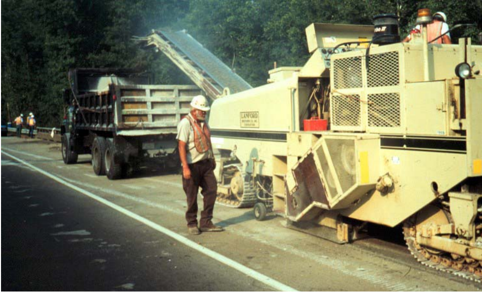
Fig. 7 Milling is the Most Economical Way to Remove Concrete
