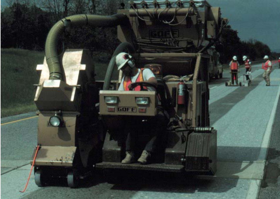
Fig. 10 Shot Blaster Cleans a 20-year Old Concrete Pavement to Provide an Excellent Surface Upon Which to Place a Concrete Overlay
