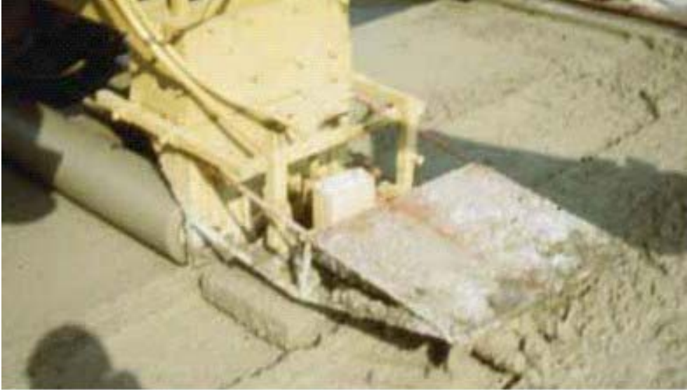
Fig. 13 The Vibrating Pan Attached to the Front of the Screed Consolidates the Overlay
