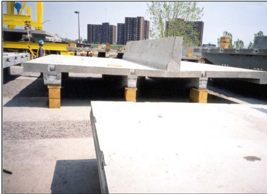
Fig. 7 Precast Prestressed Concrete Bikeway Panels
