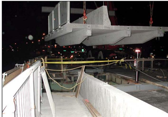
Fig. 17 Installation of New Deck Panel
