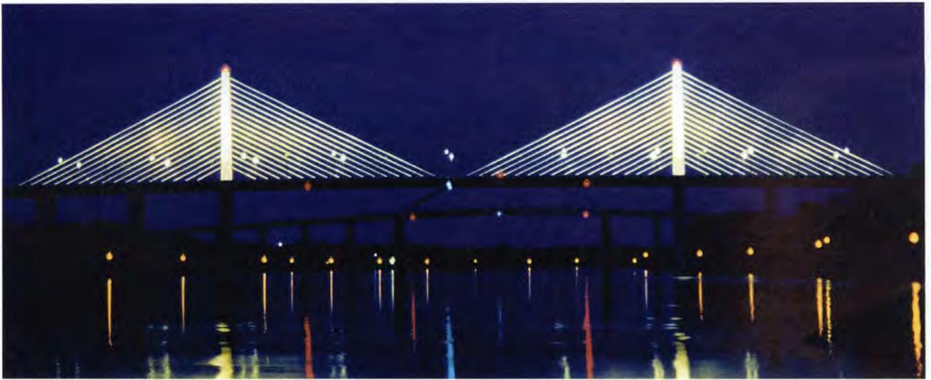
Delaware's award-winning Chesapeake & Delaware Canal cable-stayed bridge combines a dramatic visual statement with an economical design. The all-precast segmental bridge has a 750 ft (229 m) main span. Designer: Figg Engineering Group; Precast Prestressed Concrete Manufacturer: Bayshore Concrete Products Corporation.
