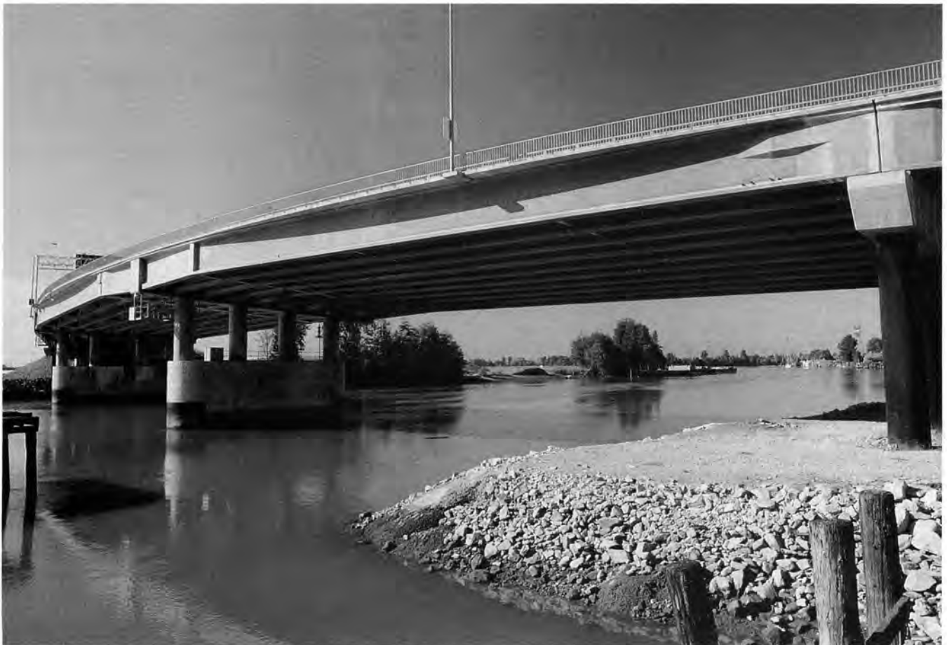
Fig. 1. Annacis Channel East Bridge, British Columbia, Canada.
