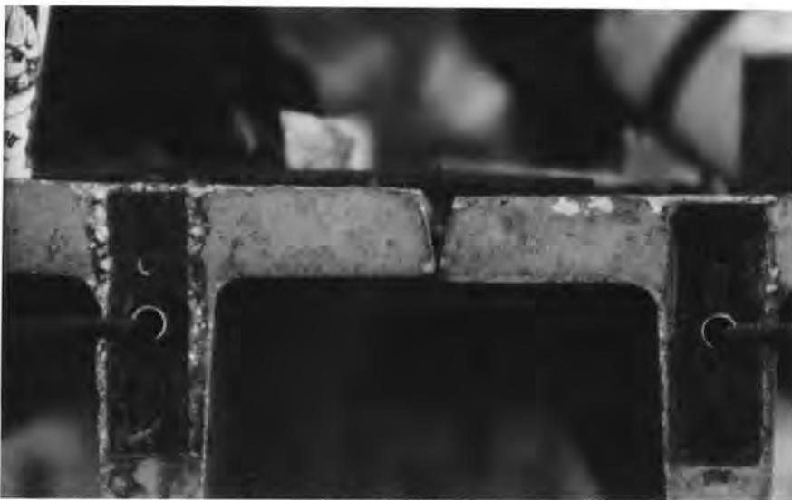
Fig. 10a. Embedded end plates and the V joint between beams.
