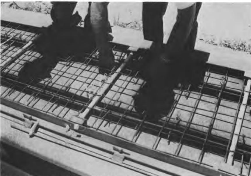
Fig. 8. Formwork of the test beam and reinforcement.
