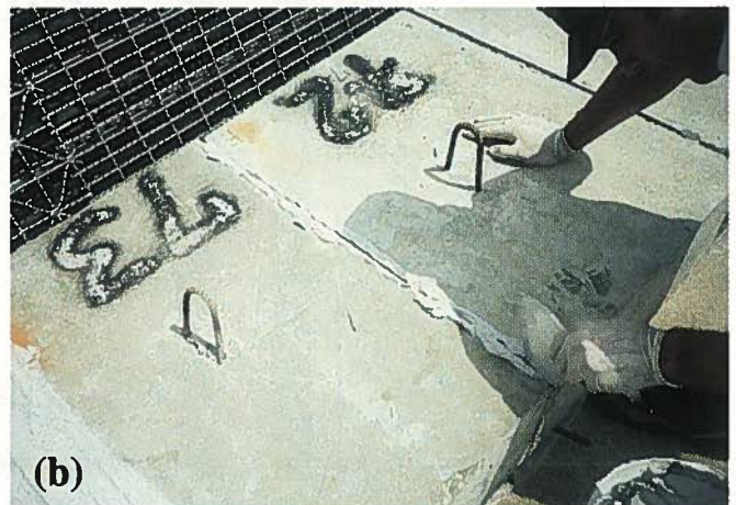
Fig. 4. Details of epoxy application: (a) Epoxy application on annulus and one face; (b) Epoxy application in a typical top strip.
