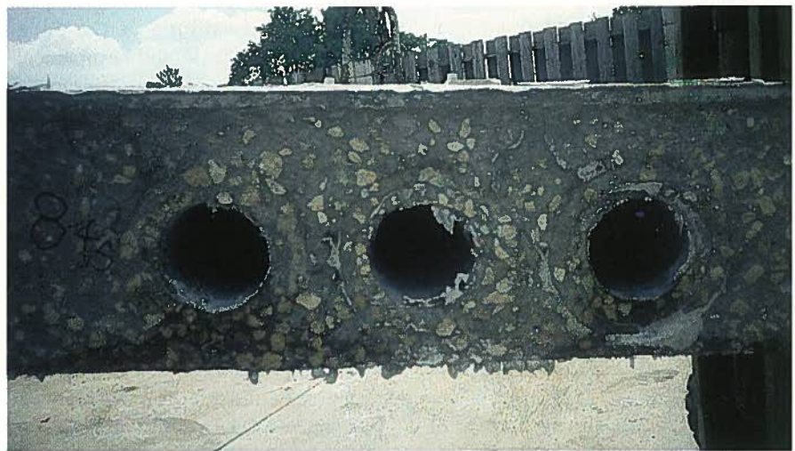
Fig. 11. Joint separation for failure test.
