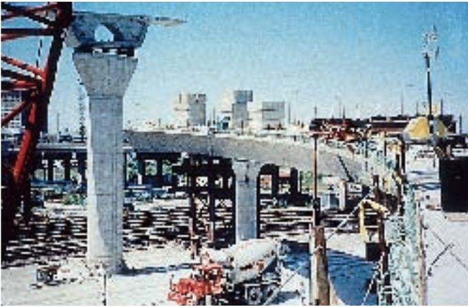
Fig. 11. Segmental concrete construction over North Station tracks.
