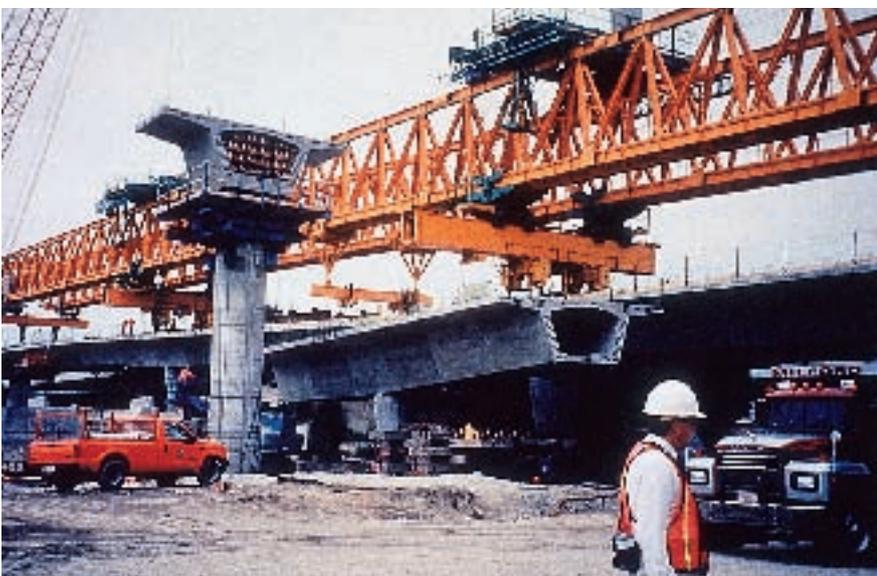
Fig. 3. Precast segmental erection.
