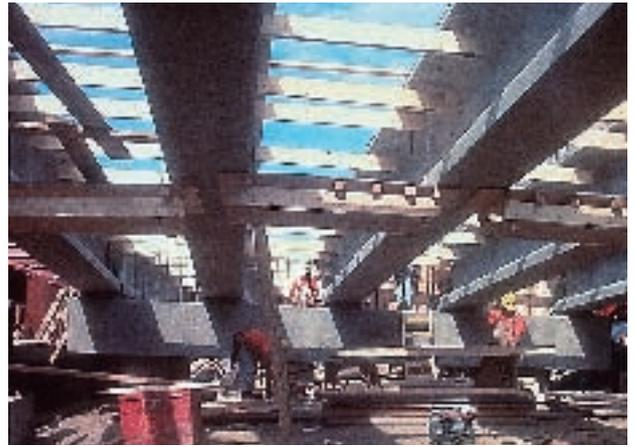
Fig. 12. New England bulb-tee girder construction.
