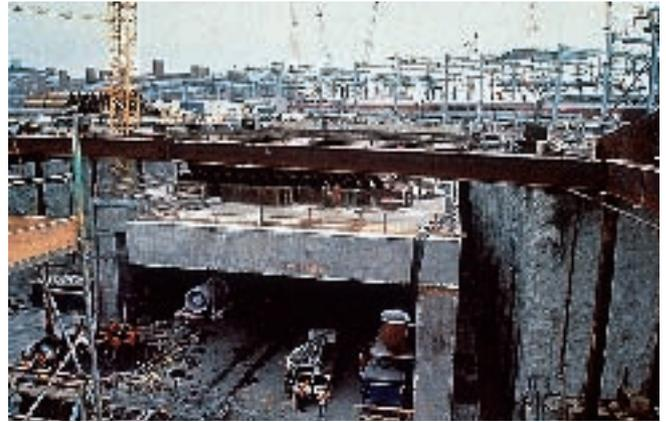
Fig. 5. Precast tunnel jacking.
