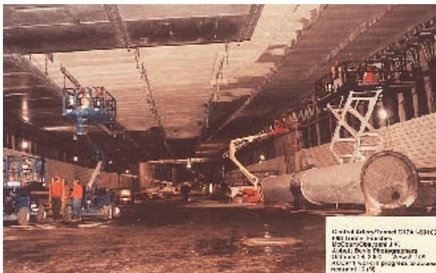
Fig. 9. Precast concrete walls and ceiling being installed.
