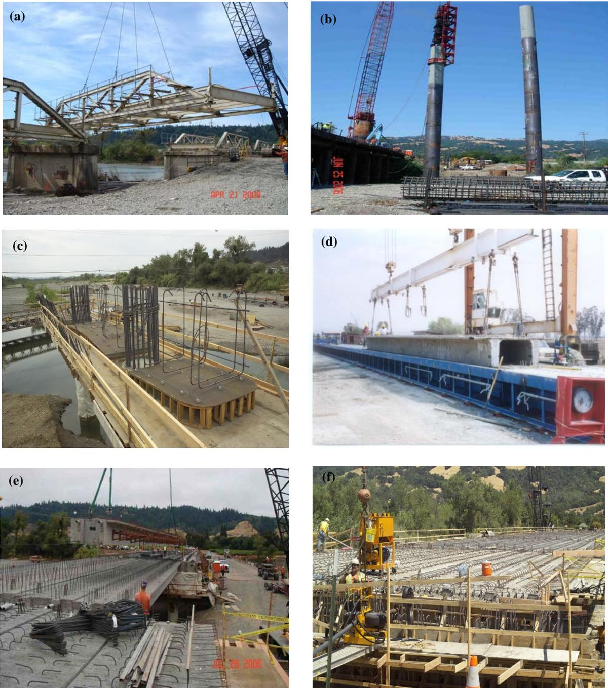
Fig. 10: Construction of the Russian River Bridge: a) Demolition of Existing Truss Bridge, b) Driving of Cast In Steel Shells, c) Forming Drop Bent Cap with Architectural Features, d) Fabrication of Double Tee Girders, e) Erection of Girders and Deck Slab Reinforcement, f) Post-tensioning – First Stage.
