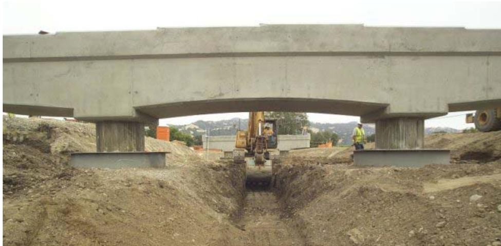
Fig. 4 Isolation of Shorter Columns at Bents 2 and 10.
