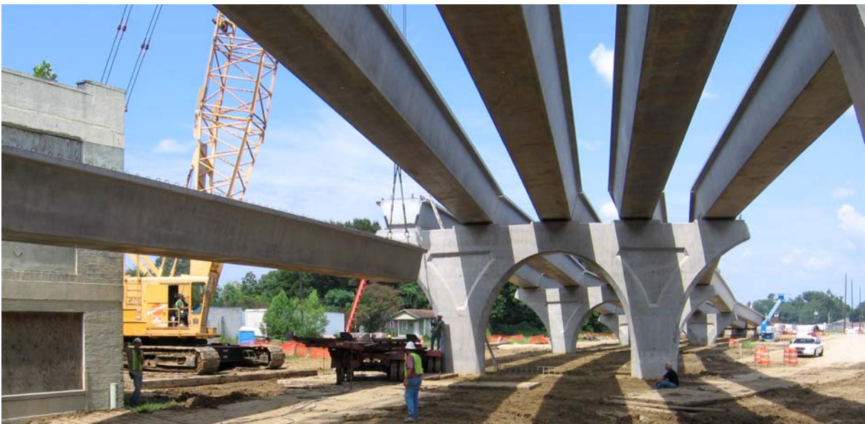
Figure 7: Precast Prestressed Concrete Box Girders Erected
