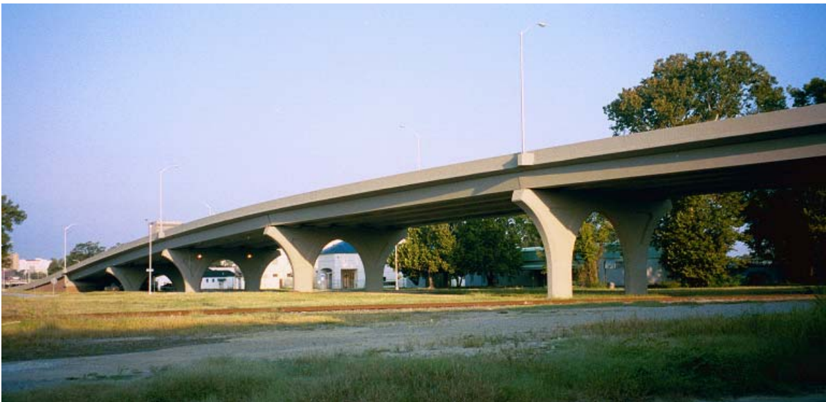
Figure 1: Finished Bridge Elevation View of the West Spans
