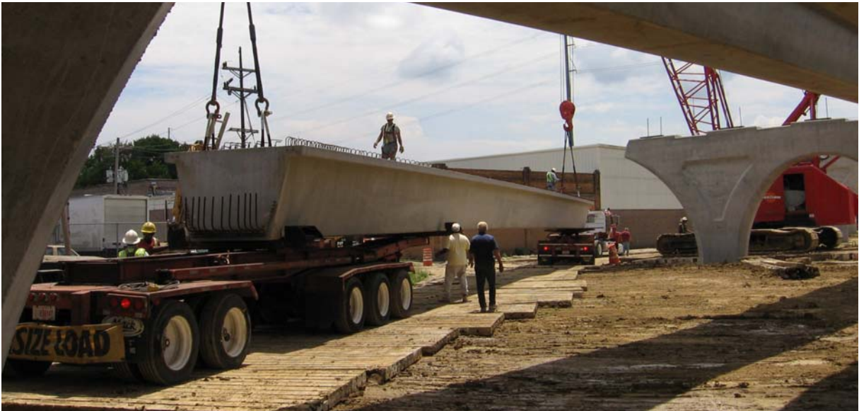
Figure 6: Precast Prestressed Concrete Box Girder Delivered by Trucks
