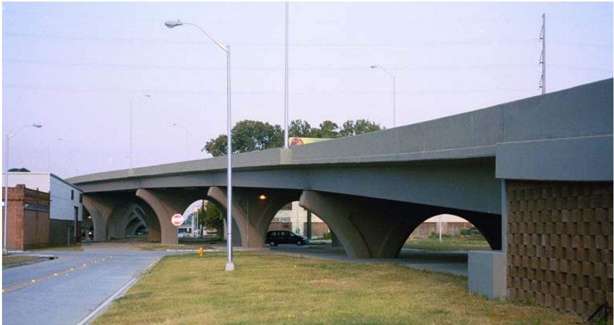
Figure 2: Finished Bridge Elevation View of the East Spans
