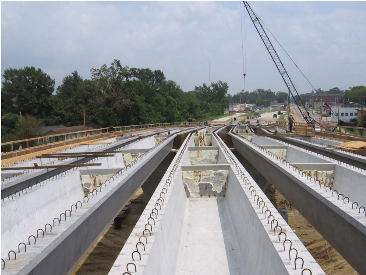
Figure 8: Precast Prestressed Concrete Box Girders Erected
