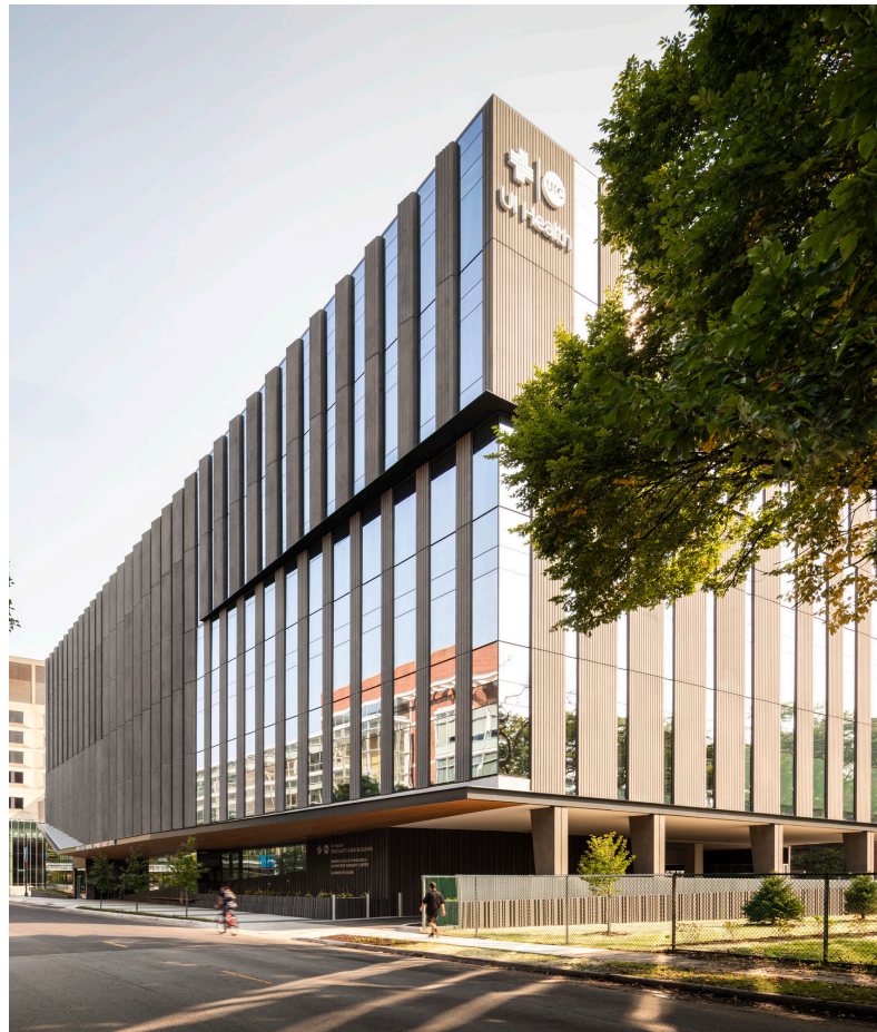
The University of Illinois Health Specialty Care Building, a new outpatient surgery center in the heart of Chicago’s Medical District, is a six-level, 200,000 ft 2 (19,000 m 2 ) facility that includes two levels of same-day surgery suites, three levels of specialty clinics, and a ground floor with check-in, pharmacy, and imaging services. Courtesy of AJ Brown Imaging.
