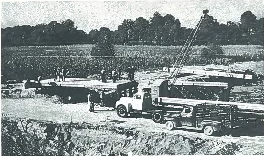
Fig. 10a. Erection of block-beams hauled 176 miles from fabricating plant to erection site, Obion County, Tennessee (about 1950).
