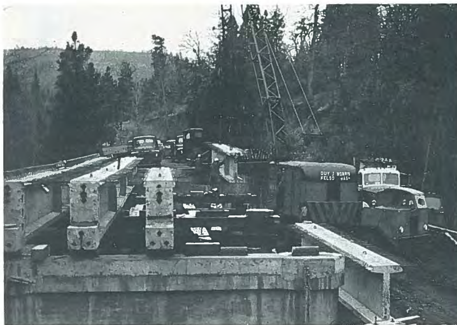
Fig. 78. Girder sections being erected on falsework at site.
