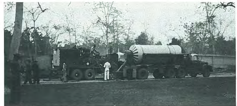
Fig. 11. Halliburton grouting the girders.
