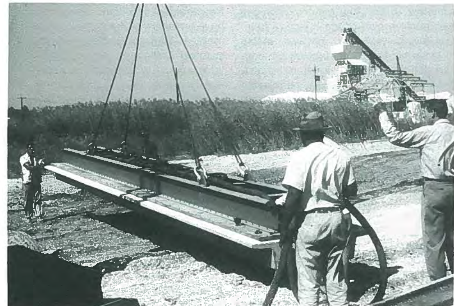
Fig. 14. Vacuum lifter in action raises and removes precast non-prestressed channel seats from the molds for later use in Loyola University's stadium. This structure is an early example of the combined use of prestressing with precasting techniques.
