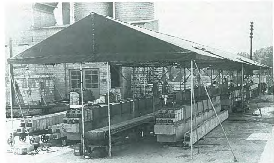
Fig. 15. Fabrication of joist for Wilkins Air Force Depot.
