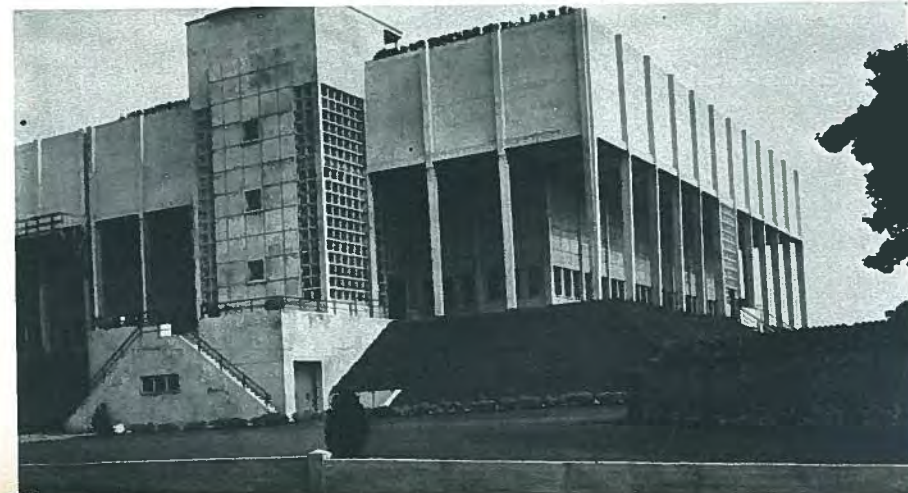
Fig. 31. Water storage reservoir and offices, Orleans, France.
