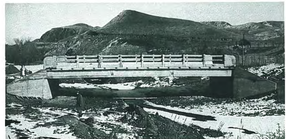
Fig. 5. The Ross Creek Bridge at Medicine Hat, Alberta, was the province's first prestressed concrete bridge (1953).
