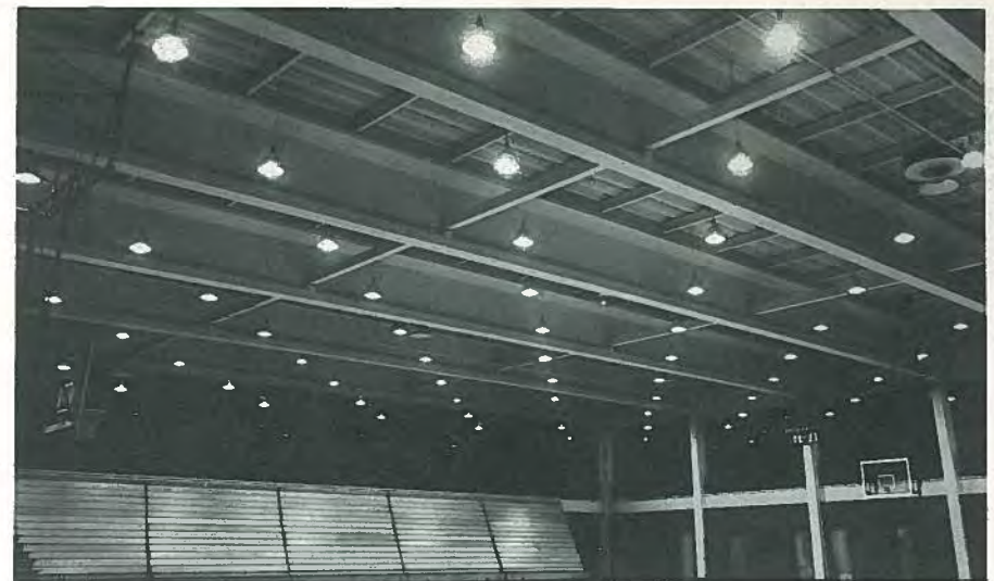
Fig. 42. Completed gymnasium with 120-ft clear span.
