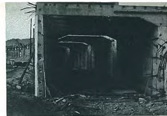
Fig. 30. Covered viaduct under construction, Rouen, France.
