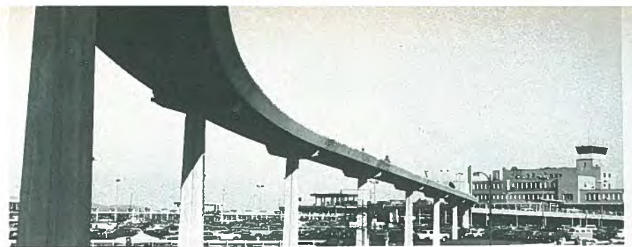
Fig. 91. View of completed Bradley Field guideway, Hartford, Connecticut.
