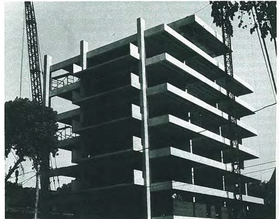
Fig. 24. Grosvenor House in Winnipeg, tallest all-precast building in Canada at the time of its construction (1960).
