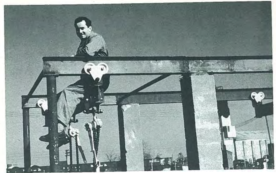
Fig. 21. Jean Muller, a welcome visitor to Prestressed Concrete of Colorado, takes a break on the support rails of the jacking assembly.
