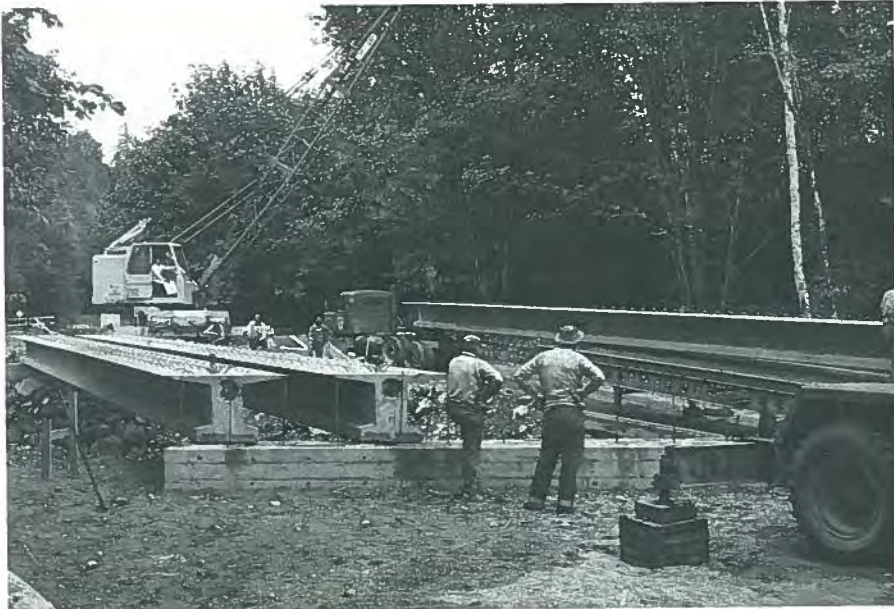
Fig. 81. Bulb T-beams being placed at erection site.
