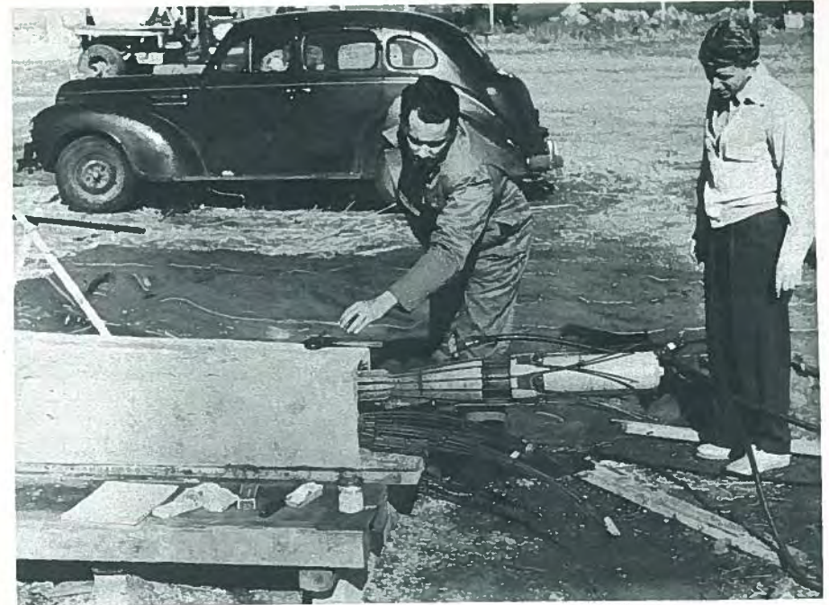
Fig. 28. Jean Muller (left) and Jack Perlmutter work together on the post-tensioning of a beam to be used with pretensioned channel slabs for Denver Livestock Feed.
