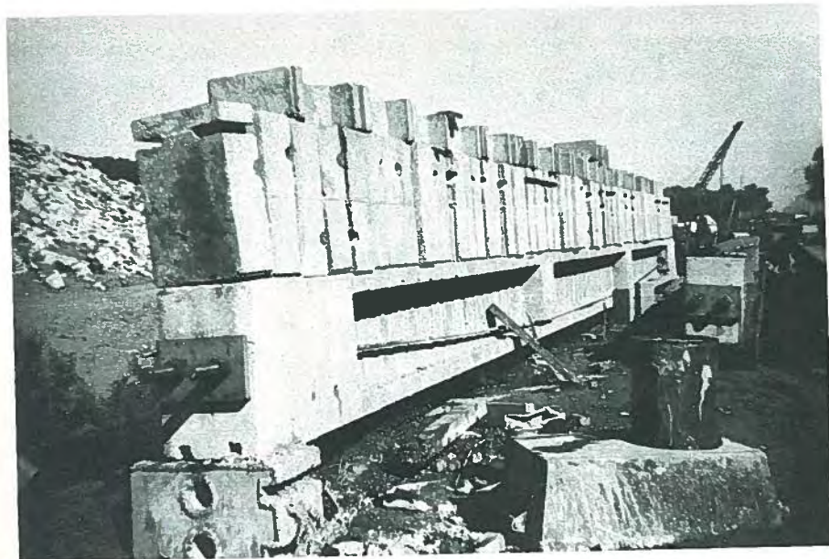
Fig. 15. Testing of Michigan block-beam with 1.5 live load.
