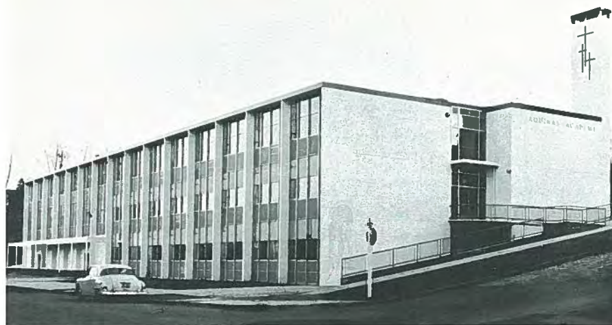
Fig. 67. Completed school, after only 6 months of construction.
